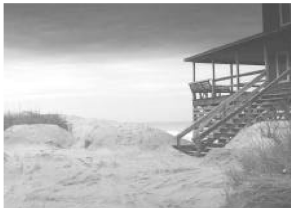
Above: The septic systems along Abram Street in South Nags Head take a beating from stormy weather and have to be monitored closely. Page 18: View of Nags Head from ocean. All photos by Todd Krafft.
