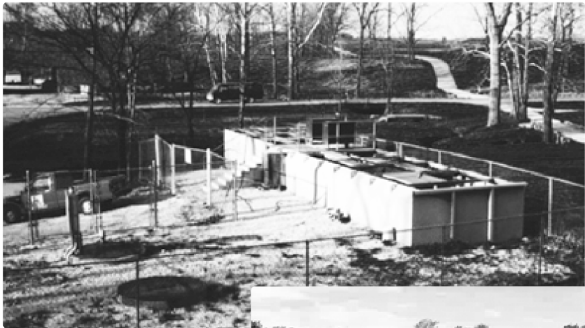
Options for small system treatment include package plants (top) and oxidation ditches (bottom). Photos courtesy of Lorene Lindsey.
