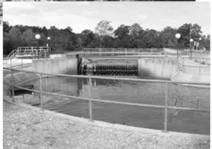
Options for small system treatment include package plants (top) and oxidation ditches (bottom). Photos courtesy of Lorene Lindsey.
