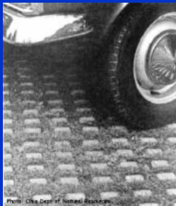
Porous design minimizes impervious area
