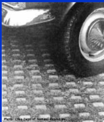
Porous design minimizes impervious area
