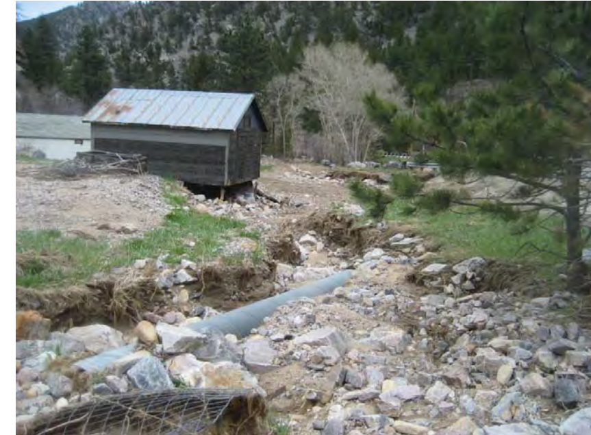
Photo 20 – Culvert conveying water in front of structures to the creek; currently partially filled with debris
