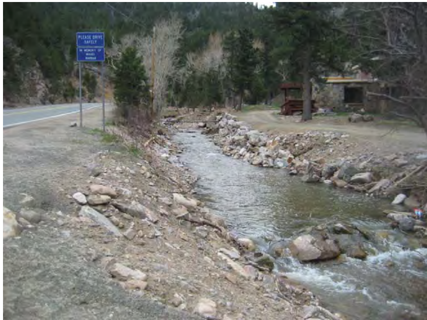
Photo 18 – Reconstructed channel, with riprap stabilizing the left bank
