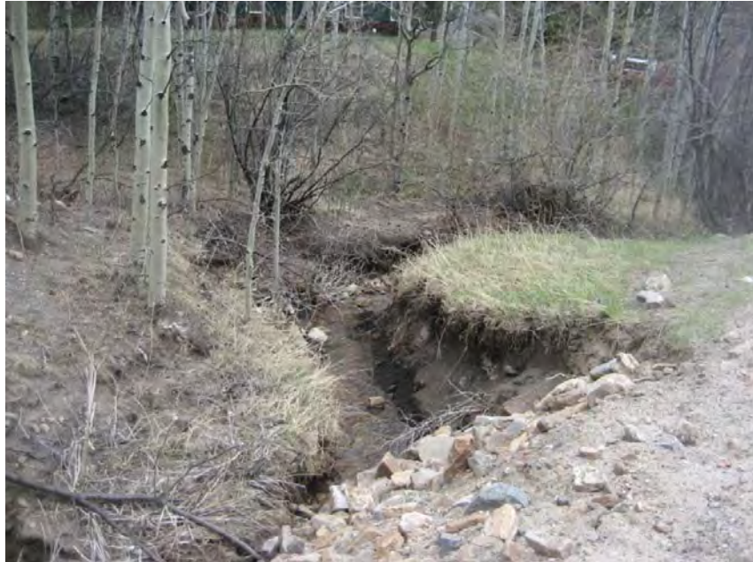
Photo 47 – Immediately downstream of the culvert, banks have been undermined
