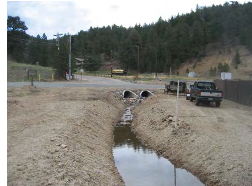
Photo 39 – New culverts under the highway and channel leading to Coal Creek
