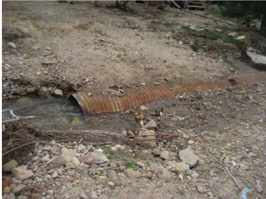
Photo 44 – Culvert already near its capacity, even with relatively low flows
