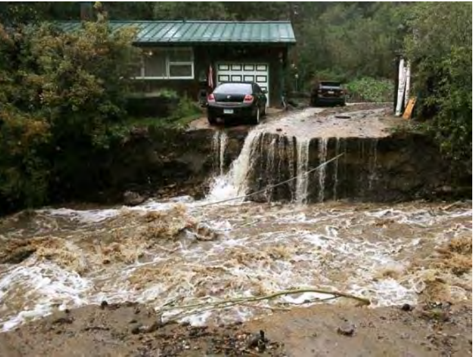
Photo 2 – Driveway Culvert Failure on Coal Creek
