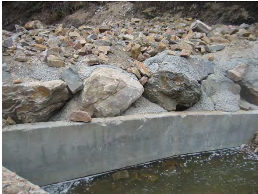
Photo 22 – Grouted riprap added to upstream end of box culvert since the flood event
