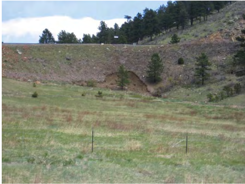
Photo 1 – Scouring of the railroad's south bank
