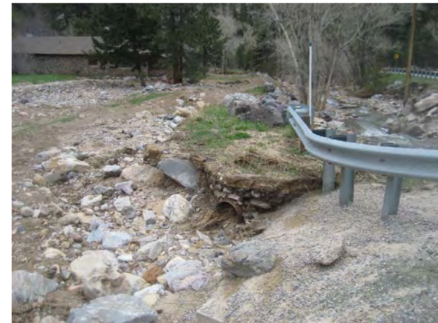
Photo 20 – Culvert conveying water in front of structures to the creek; currently partially filled with debris
