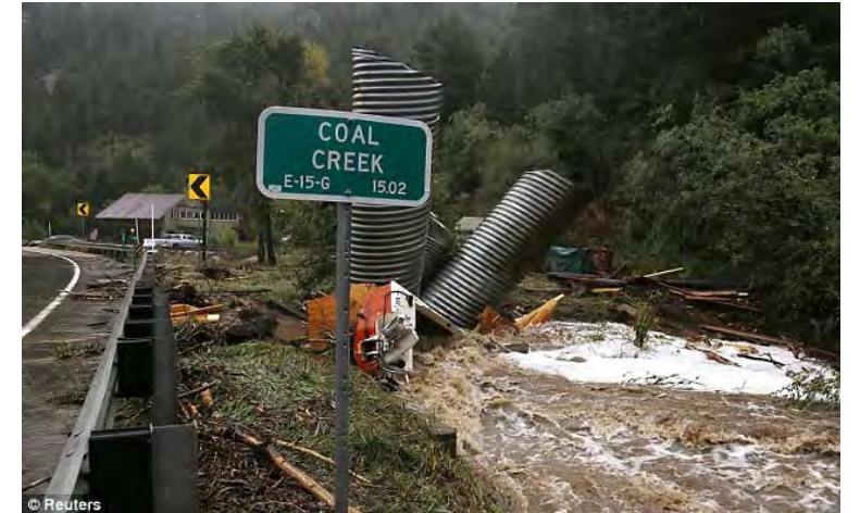
Photo 10 – Debris within Coal Creek due to Sediment Flows
