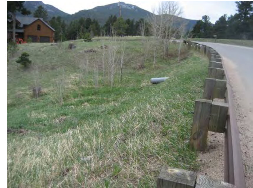
Photo 52 – Culvert passing under Crescent Park Drive
