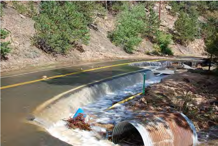
Photo 5 – Highway Inundation at Twin Spruce Gap Road
