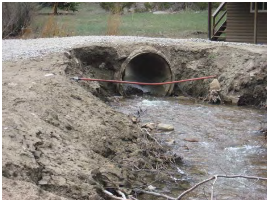
Photo 48 – Undermined culvert on Beaver Creek
