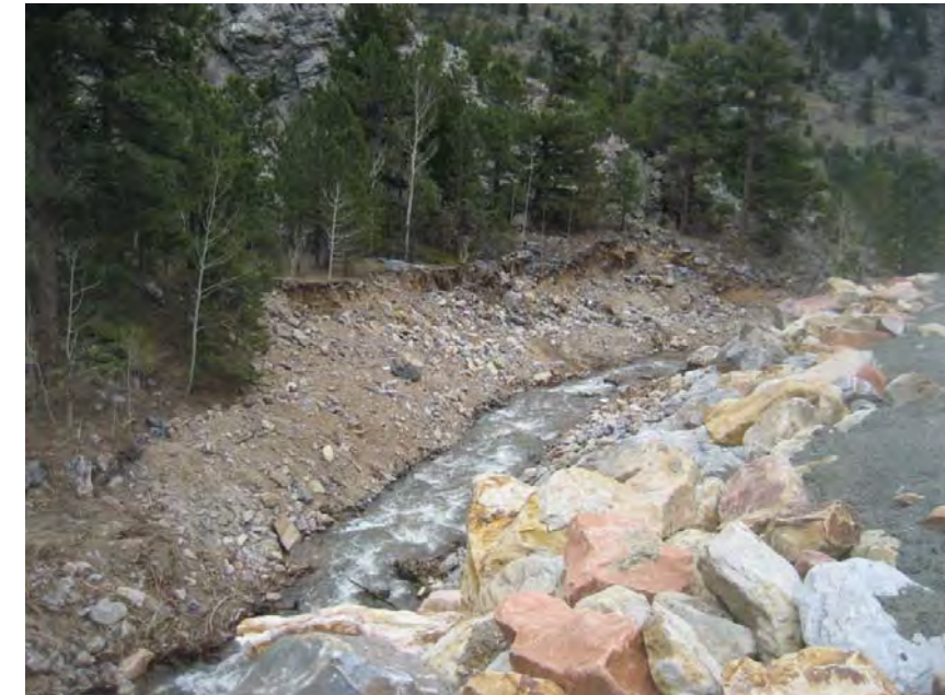
Photo 13 – Severely scoured left channel bank, and newly constructed right channel bank
