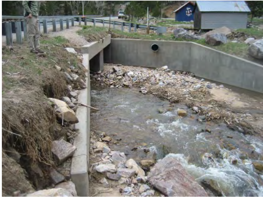
Photo 22 – Grouted riprap added to upstream end of box culvert since the flood event
