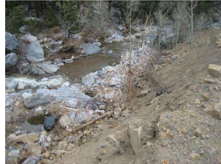
Photo 16 – Exposed dirt on right channel bank abutting the highway
