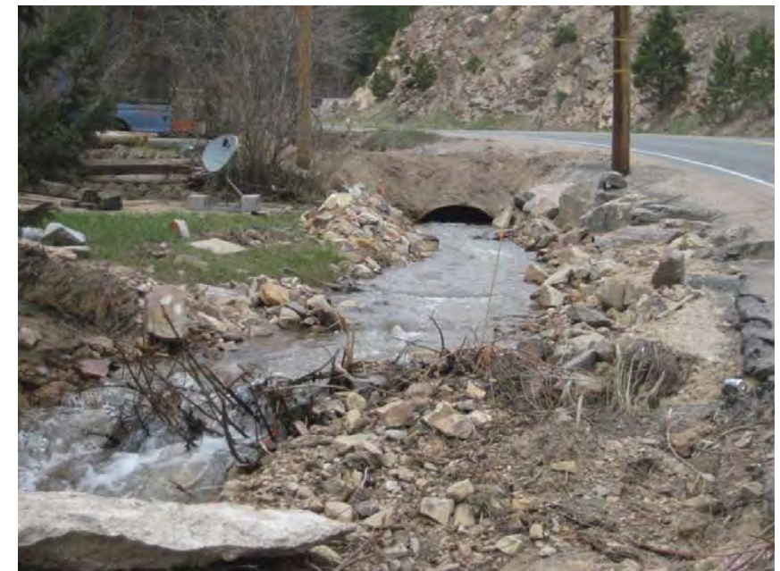
Photo 43 – Newly installed culvert under driveway, seemingly undersized; debris in overbank
