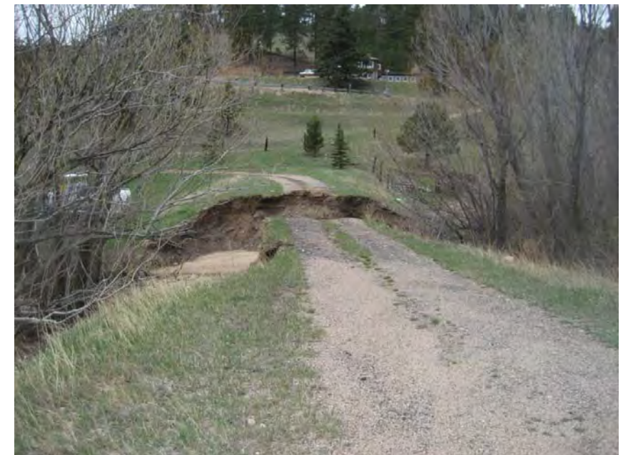
Photo 36 – Destroyed roadway formerly crossing the creek
