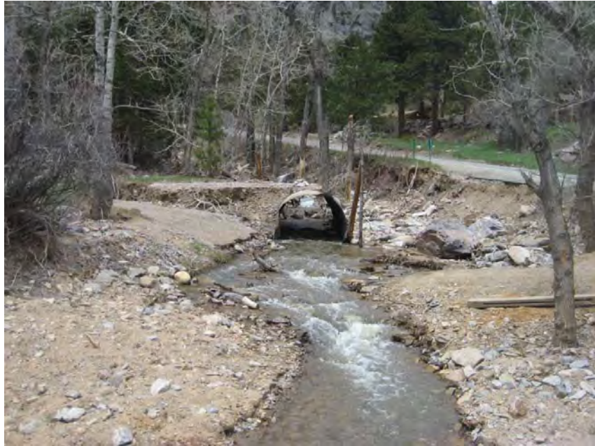
Photo 26 – New driveway and culverts installed at one residential structure
