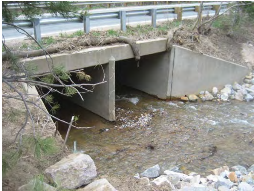
Photo 8 – Upstream entrance to box culvert under highway
