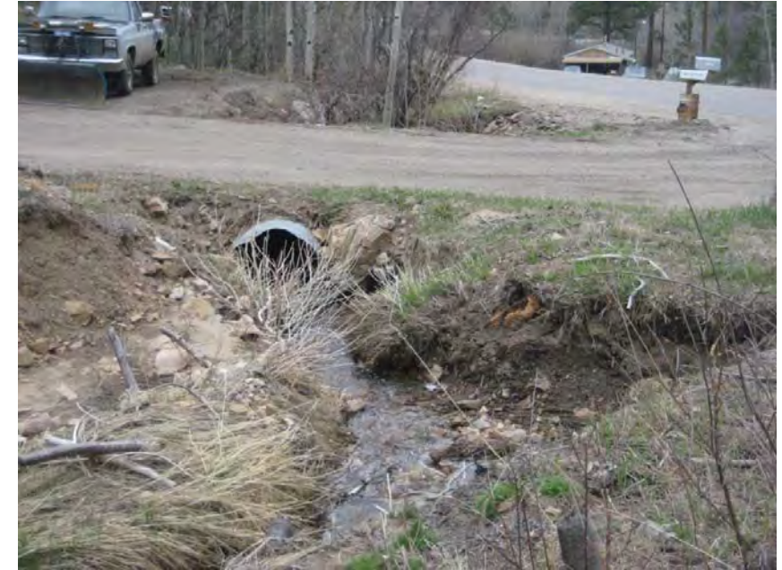
Photo 46 – Downstream end of the culvert, where the bank has eroded away
