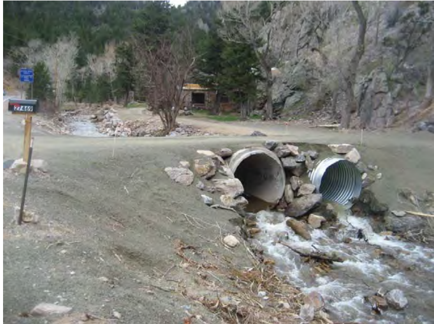
Photo 18 – Reconstructed channel, with riprap stabilizing the left bank
