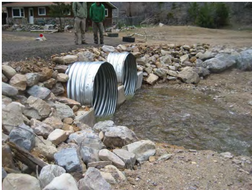
Photo 26 – New driveway and culverts installed at one residential structure
