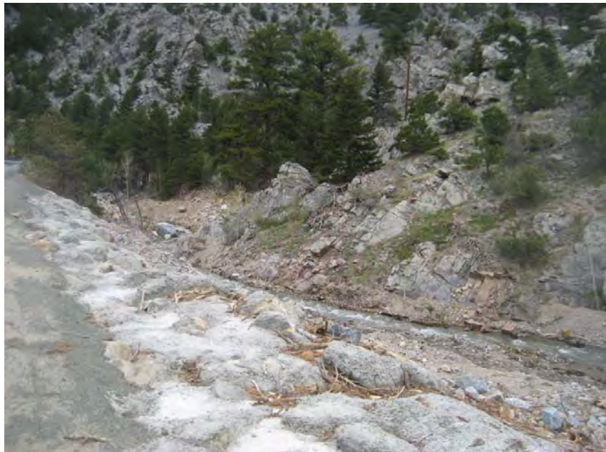
Photo 12 – Freshly installed grouted riprap between creek and highway
