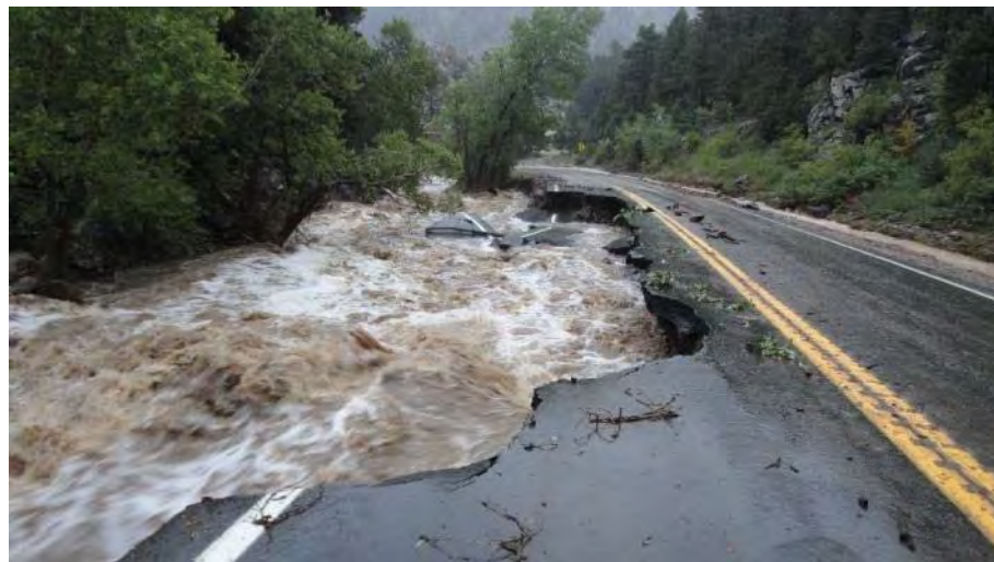
Photo 3 – One of Numerous Washouts along Highway 72
