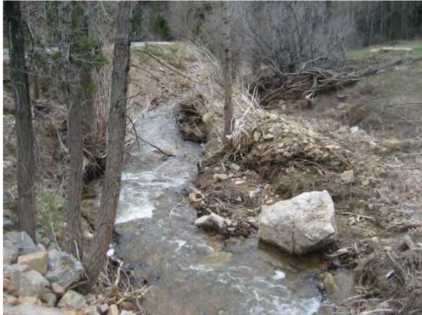
Photo 33 – Accumulated debris along overbanks
