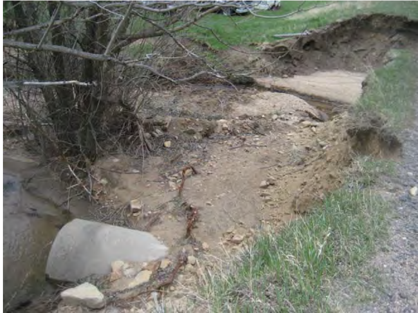
Photo 37 – Sand deposition in the channel; culvert mostly filled with sediment
