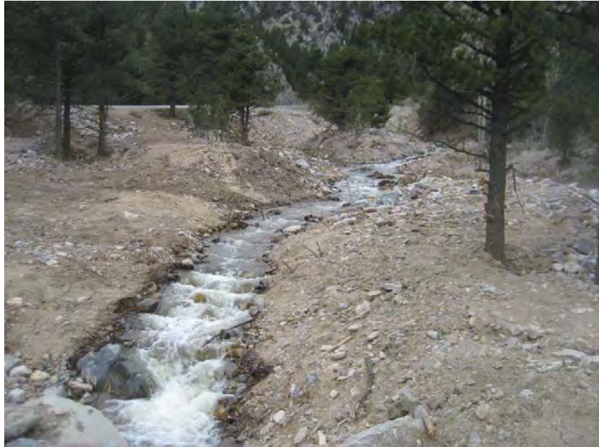
Photo 11 – Reconstructed creek downstream of culverts
