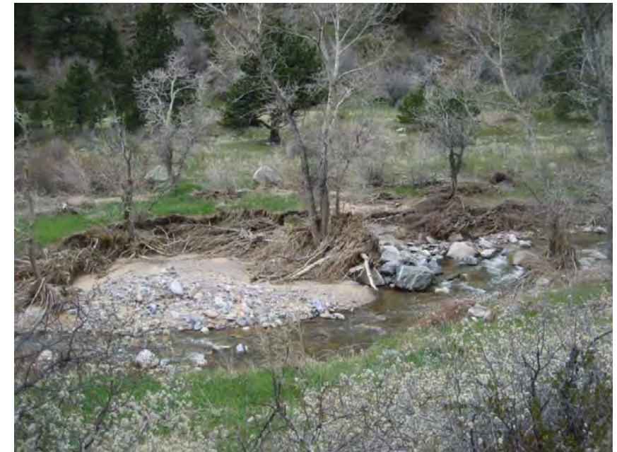
Photo 3 – Scouring of the creek's right bank
