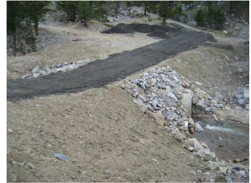
Photo 10 – Reconstructed creek upstream of culverts
