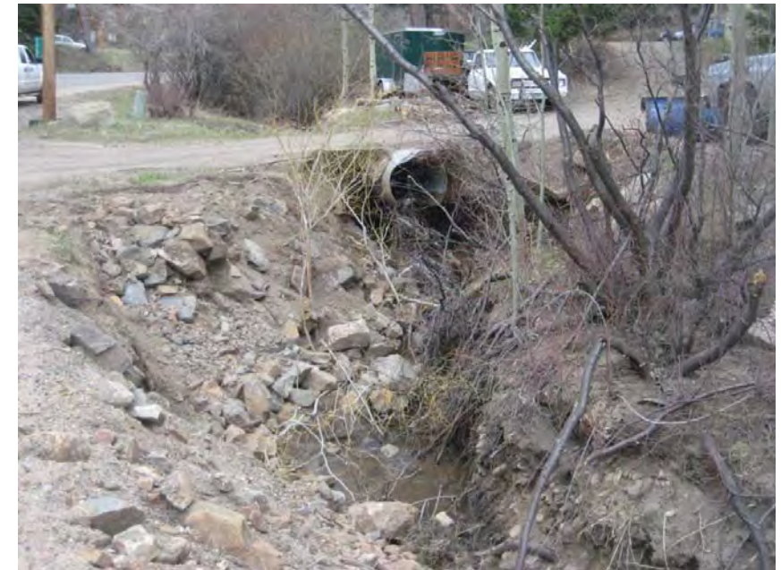
Photo 46 – Downstream end of the culvert, where the bank has eroded away
