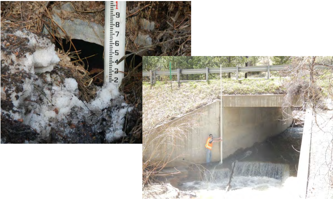
Photo 4 – Culverts range from small and mostly blocked to large box culvert roadway crossings
