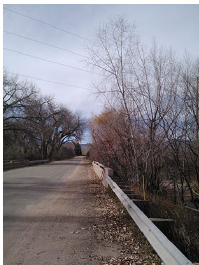
LH-13A LOOKING WEST
