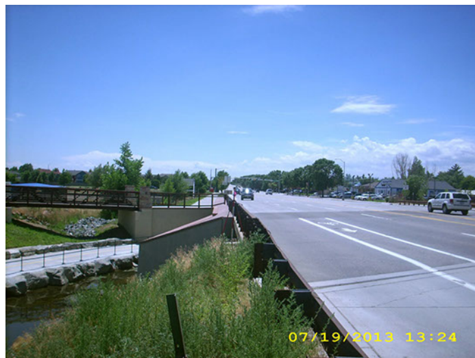
L.H. NO.2 LOOKING SOUTH
