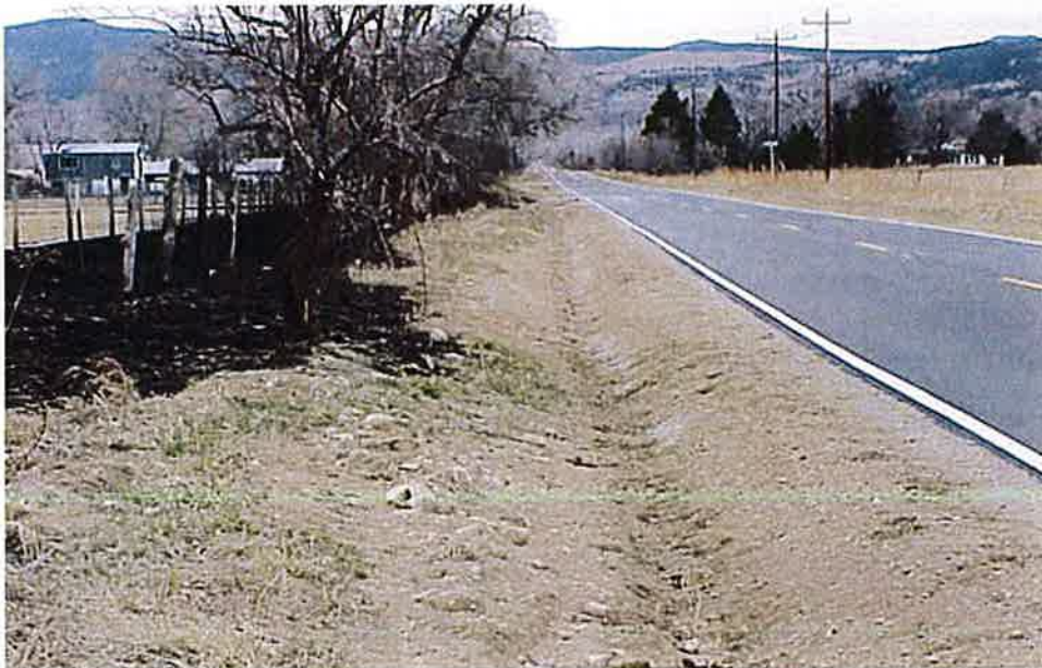
Figure 900-3. Example of a Roadside Ditch (Boulder County, 2016).
