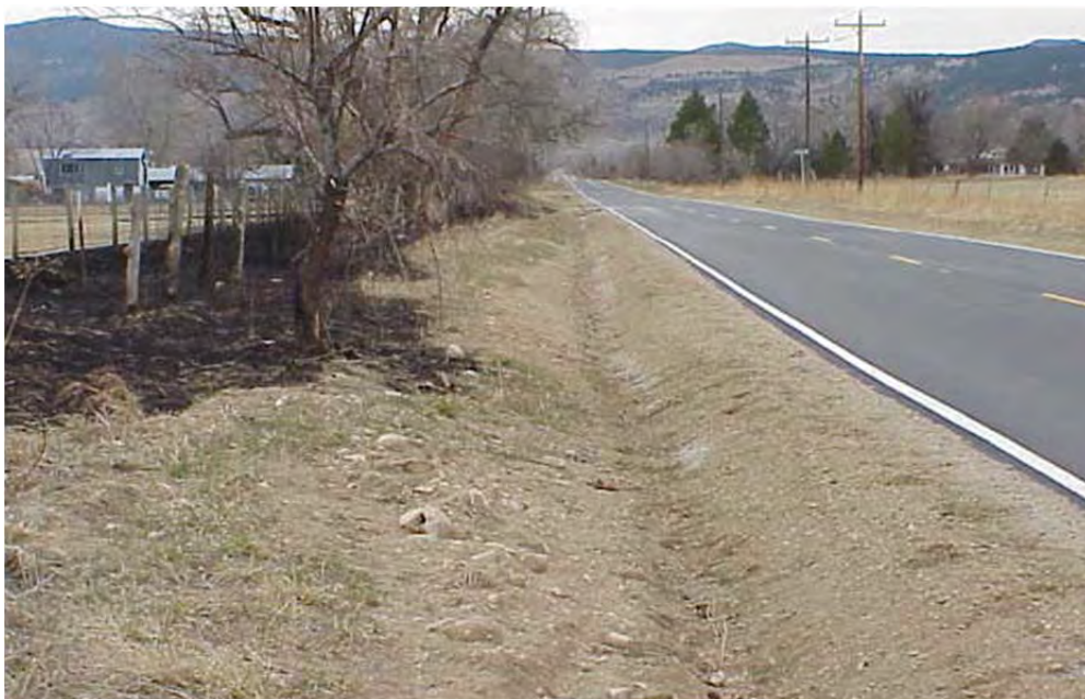
Figure 900-3. Example of a Roadside Ditch (Boulder County, 2016).
