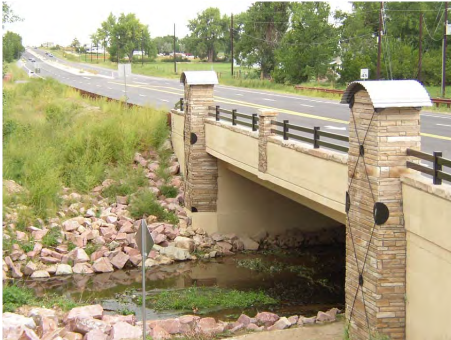
Figure 1000-3. Example of a Bridge With an Aesthetic Component (Boulder County, 2016).
