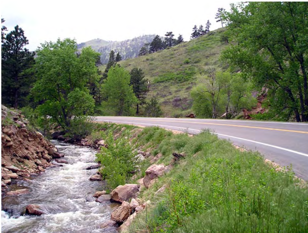
Figure 900-4. Example of a Roadway Adjacent to a Channel (Boulder County, 2016).
