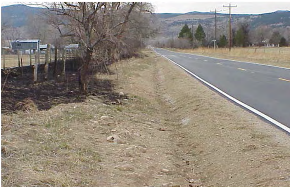
Figure 900-3. Example of a Roadside Ditch (Boulder County, 2016).
