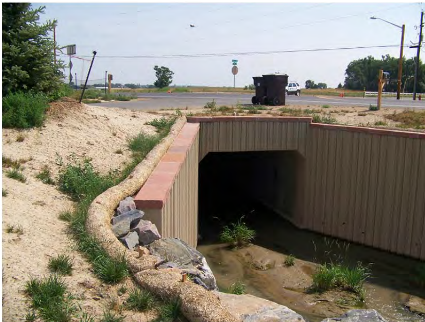
Figure 1000-1. Example of a Concrete Box Culvert Adjacent to a Trail (Boulder County, 2016).
