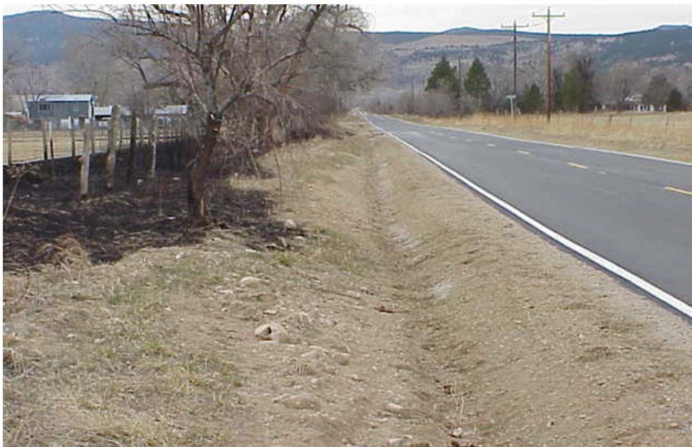
Figure 900-3. Example of a Roadside Ditch (Boulder County, 2016).
