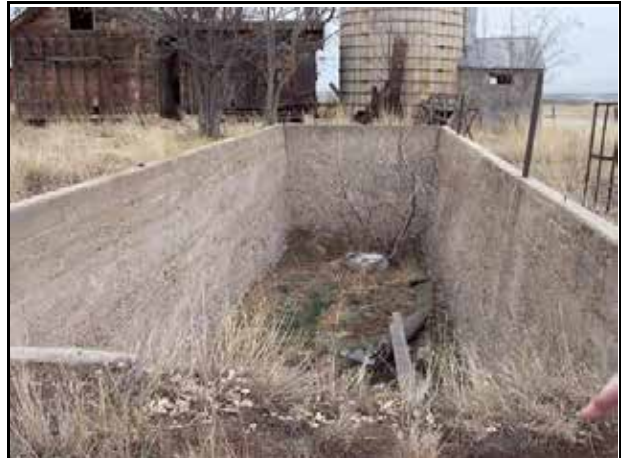
Harney Lastoka pit/trench silo. Photo by Carol Beam, BCPOS.
