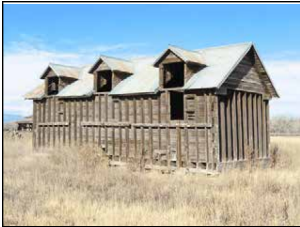
A rare studs-out granary with dormers, which were used for filling the building with grain. Photo by Carol Beam, BCPOS.
