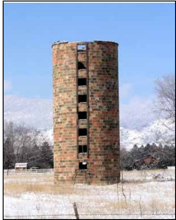
Hollow glazed clay tile silo
