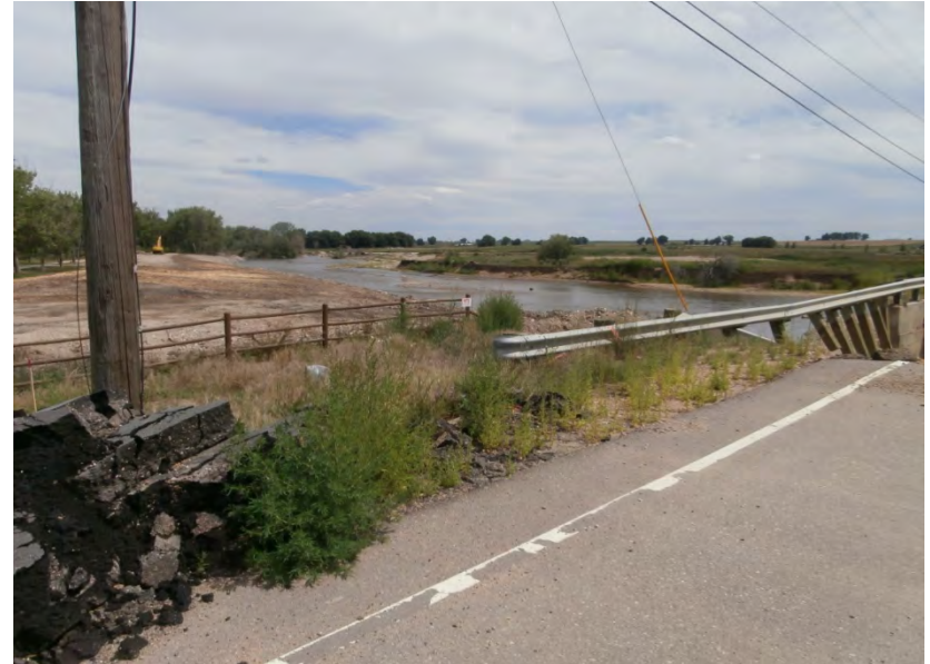
2014: View to southwest across upper channel from County Line Road. Note post-flood channel is relocated the south and pre-flood channel is barely visible to the right of the track hoe on river left.
