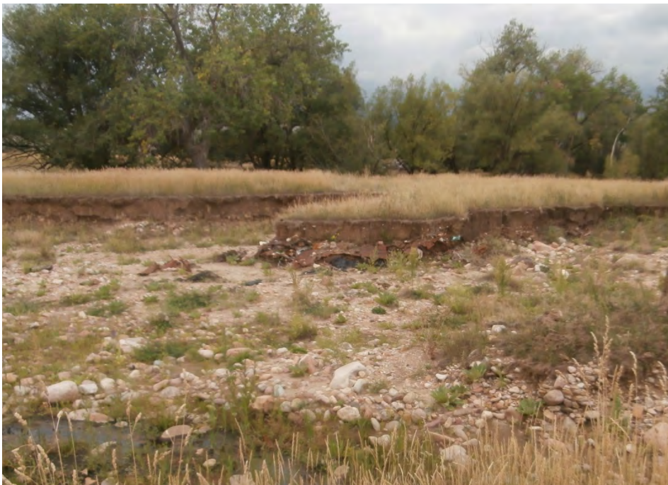
View to NW of side channels cut into river left by overland flows. Flows were approximately from photo right to photo left. Note layer of trash in center of photograph.
