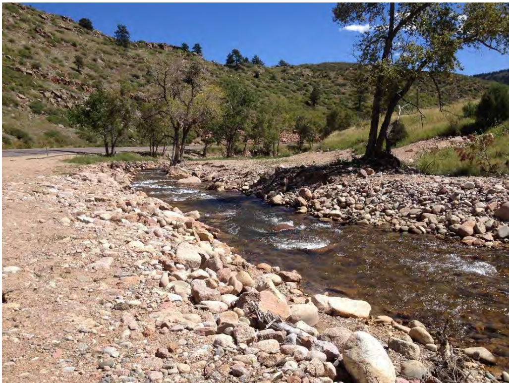
View downstream of river in graded channel of former flows. Note proximity of road to creek.
