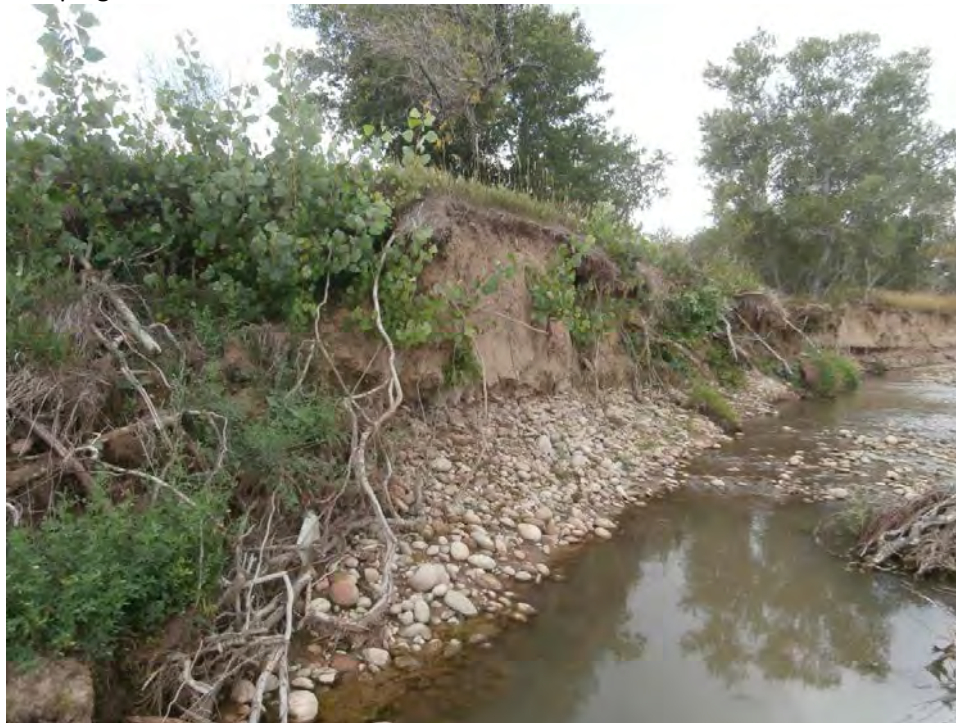
View upstream of eroded bank. Note cottonwoods resprouting from root stock in the upper soils of the bank which overlies a lower layer of very cobbly soil.
