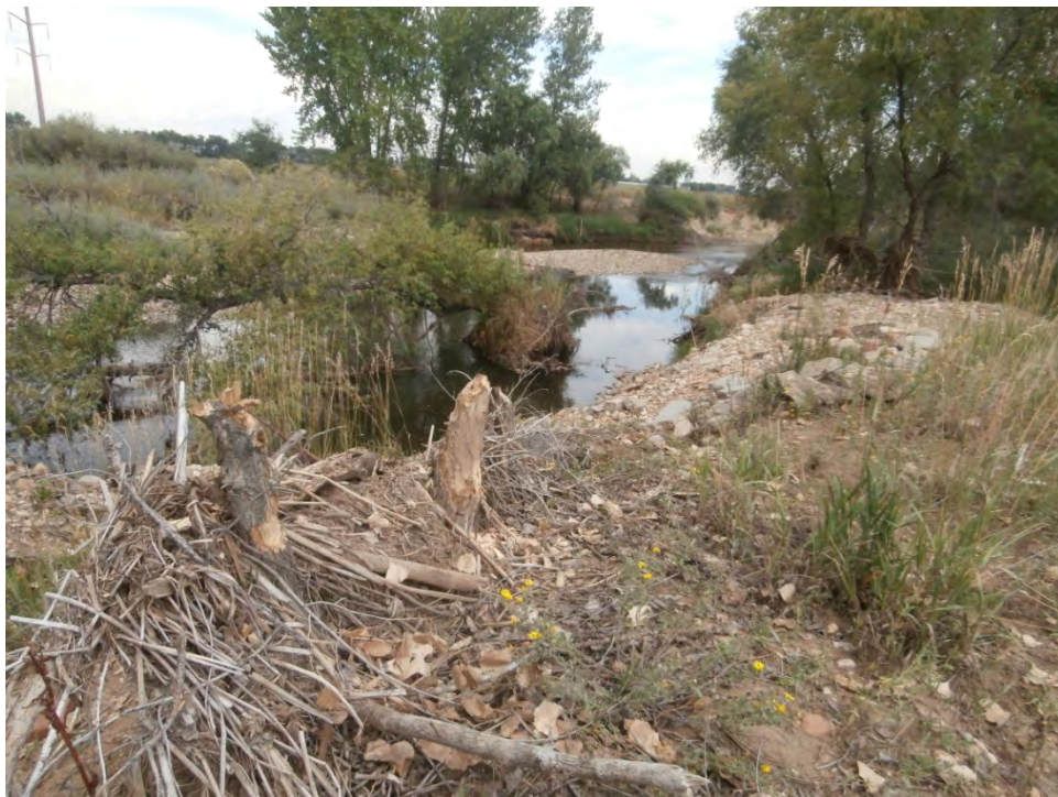
View to downstream of tree stumps left from post-flood beaver activity near lower end of property. Note bank tree, now fallen into the creek.
