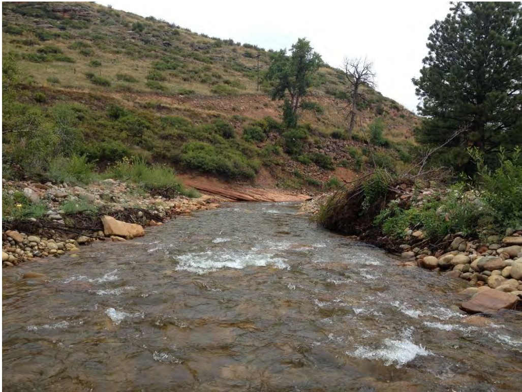
View downstream from upper boundary. Note river left bank scour and SH 7 above.
