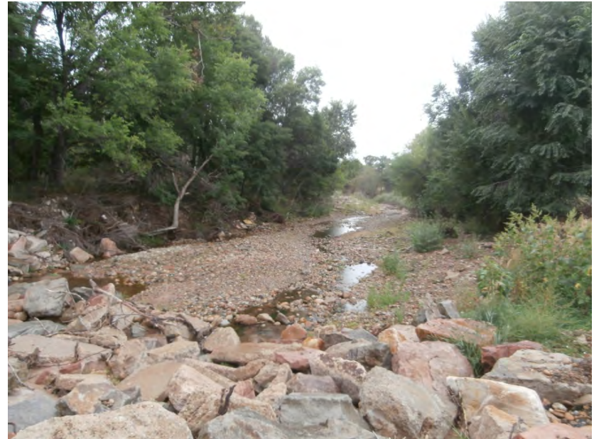
2014: View to southeast from repaired boulder dam blocking off a portion of an old channel. Note cobbly and sparsely vegetated low banks, very narrow flows.
