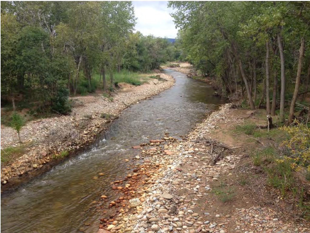
View upstream from downstream boundary. Note lack of bank vegetation.
