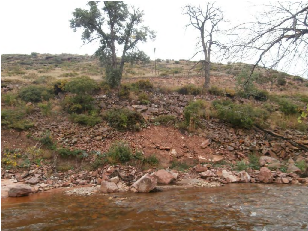
View toward SH 7 from river right (detail of previous photograph). Note potentially hazardous eroded area below highway.
