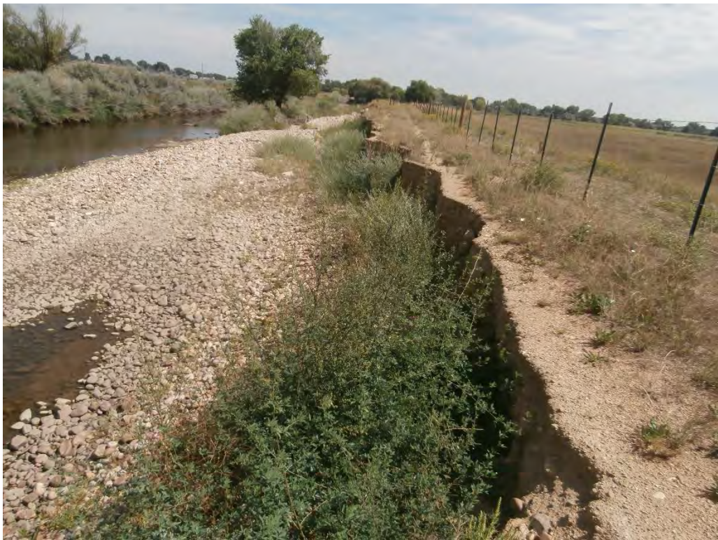
View to downstream of developing river right vegetation at toe of bank erosion. Note alfalfa in foreground and sandbar willow in background. Note intact willows on river left and remnant willow patch on river right in background.
