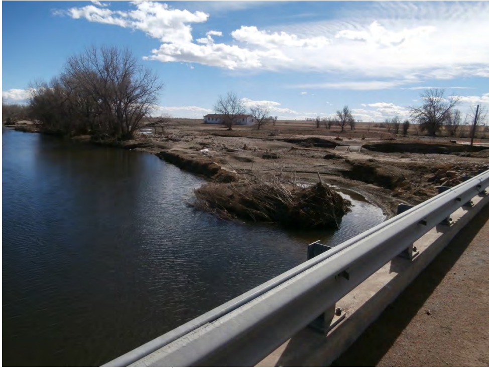
View to southeast from 119 th Street bridge on February 28, 2014. Note loss of trees; area of deposition and scour on river right.
