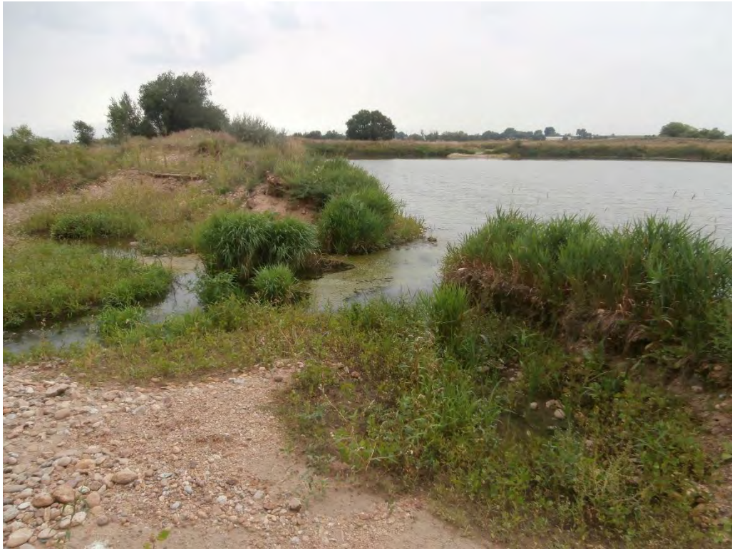
View to northwest of breach from lowest pond. Note that minor out flows continue and cottonwoods plus wetland vegetation are developing on river left upper bank.
