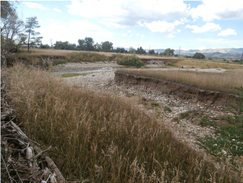
View to southwest of northern channels eroded by flood flows from breached gravel mining ponds. Note actively slumping banks in right middle ground, flows in farther channel.
