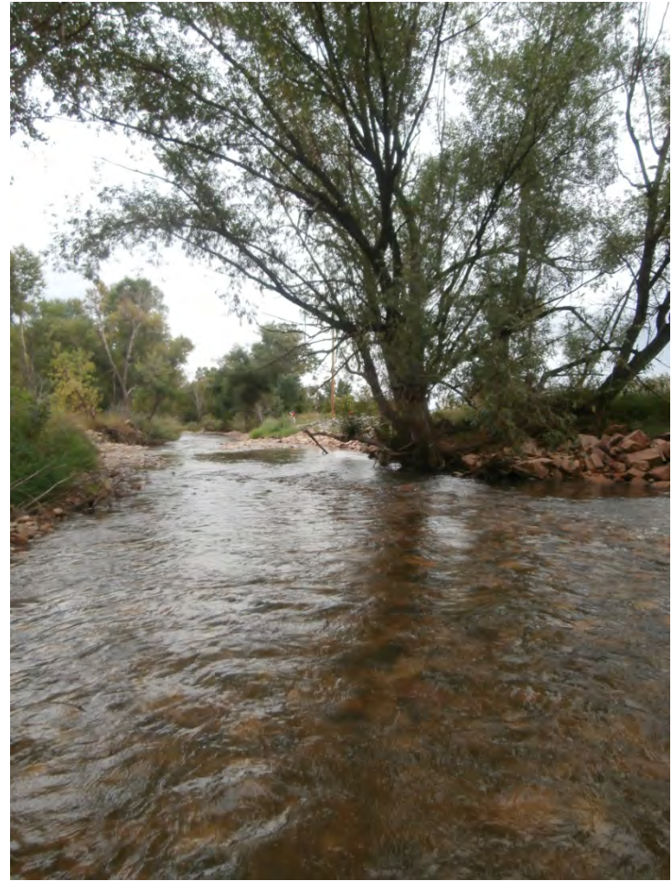
2014: View downstream from upper boundary. Note loss of branches on river right crack willow, rip rap on river right below crack willow at repair of major breach to south.
