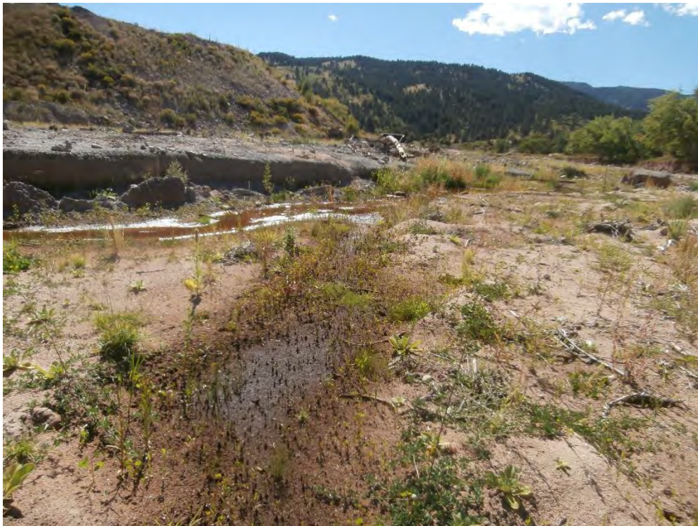
View upstream of flood path with small channel of left at toe of eroded quarry tailings. Note preferential colonization of damp areas by native woody species and presence of many weedy species in the drier areas.
