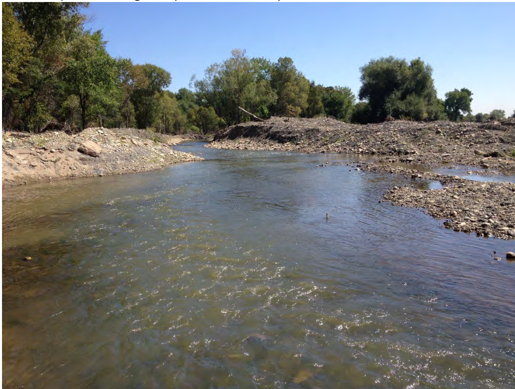
View downstream of channel work at the breach to the south.
