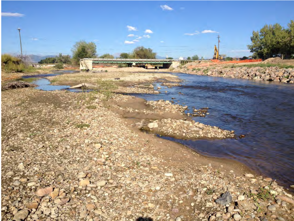
View upstream toward the damaged County Line Road bridge. Note vegetation development in foreground cobbles, new riprap bank downstream of the bridge at the right of the photograph.
