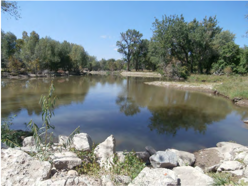
View upstream of impoundment behind irrigation structure. Note cottonwoods developing in riprap, possible crack willow at left.
