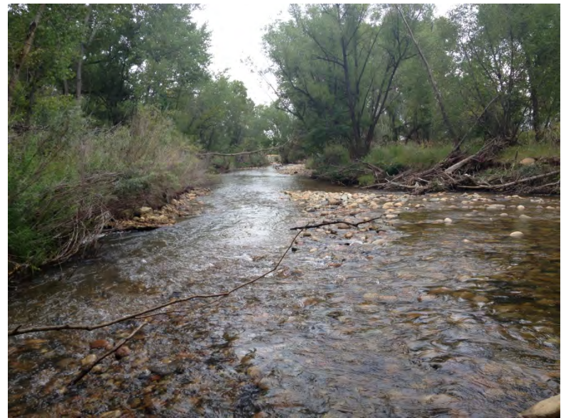
2014: View down from mid-site. Note reduction in bank vegetation and river right bank erosion and woody deposition.
