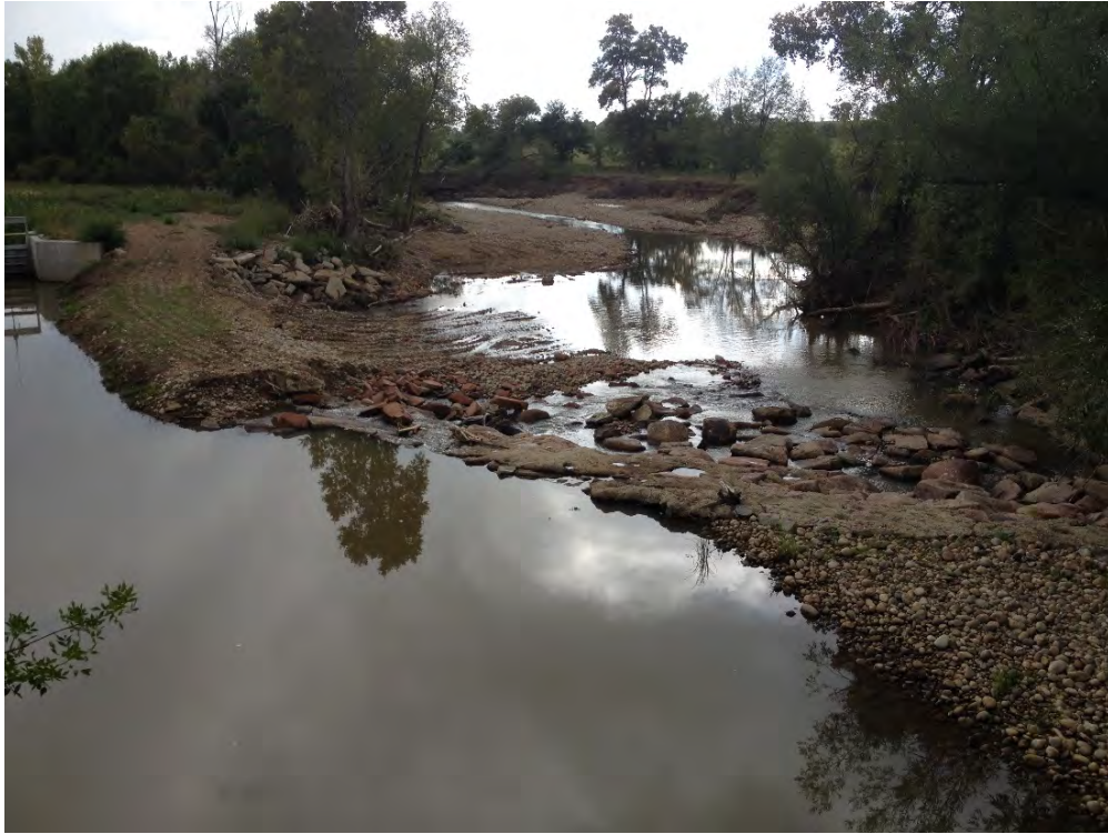
View downstream from Hygiene Road of repaired irrigation diversion structure. Note eroded banks, loss of riparian forest on river right.
