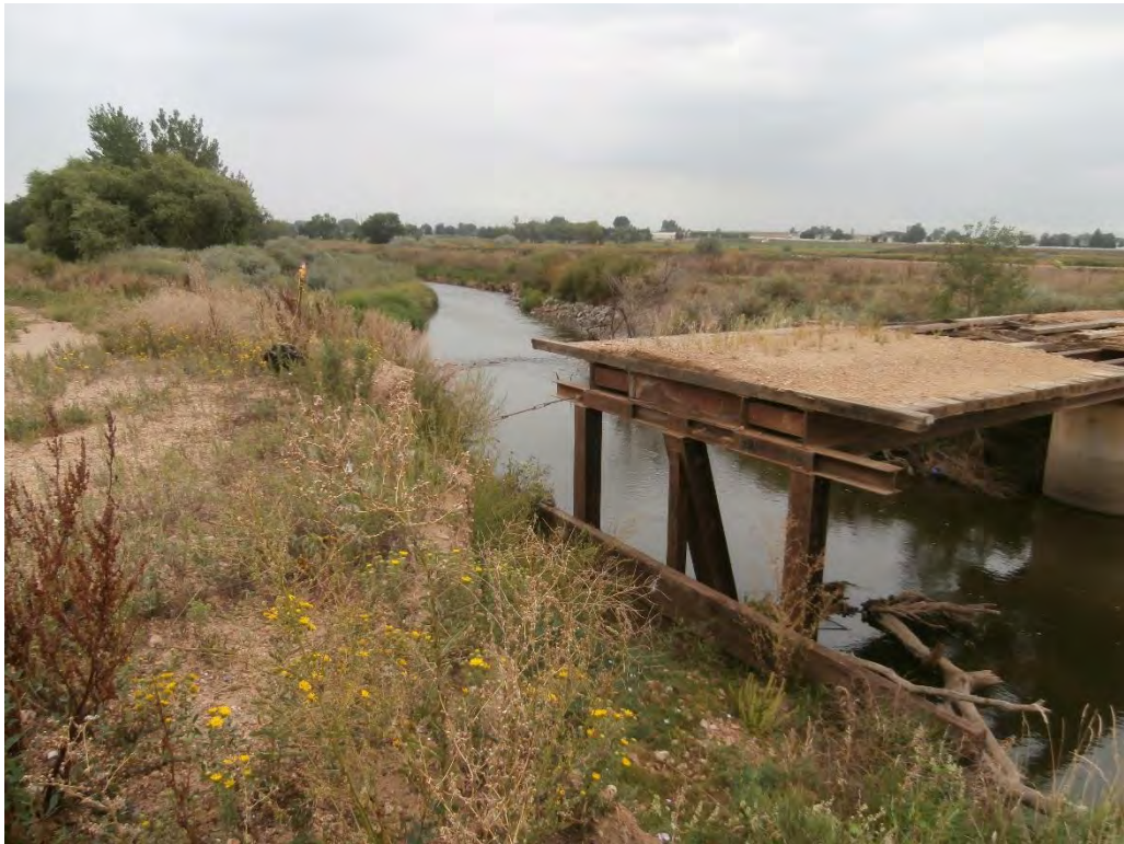
View to upstream with washed-out bridge. Note weedy foreground, intact bank willows on river left and possible tamarisk on river right.
