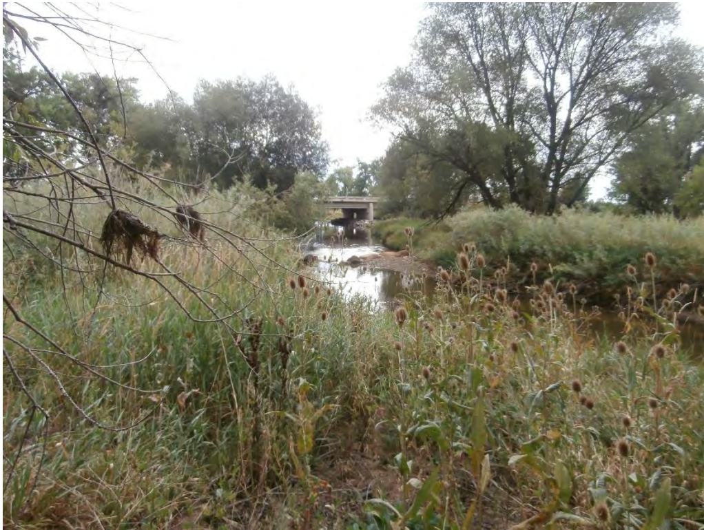
View to downstream toward US 285 bridge in background. Note teasel in foreground, flood debris on branches at left, and areas of bank willows.
