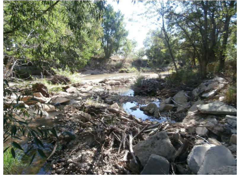
2014: View downstream from irrigation diversion. Note berm removal, foreground flood debris, eroded river left bank.
