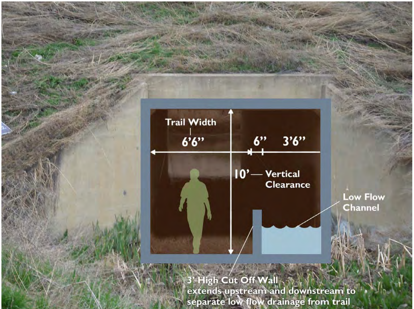
Figure 4–SH 7 Box Culvert–Alternative 1 (View Looking North) Use existing culvert for trail and low flow channel
