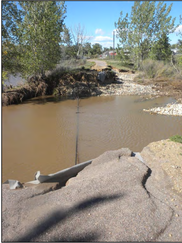
Bass Pond dam breach after flood.
