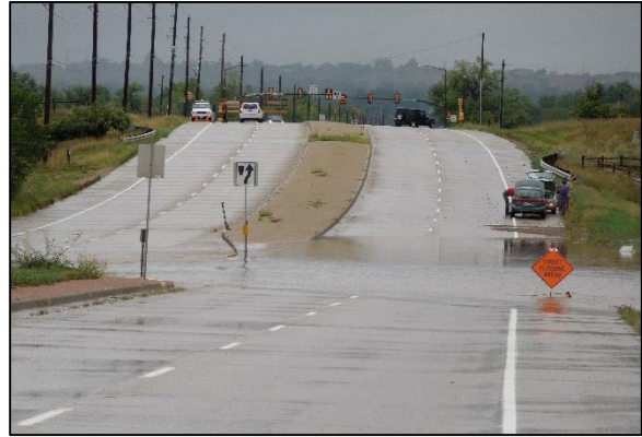
Figure 14 - South Boulder Road Overtopping Near South Boulder Creek (2013)
