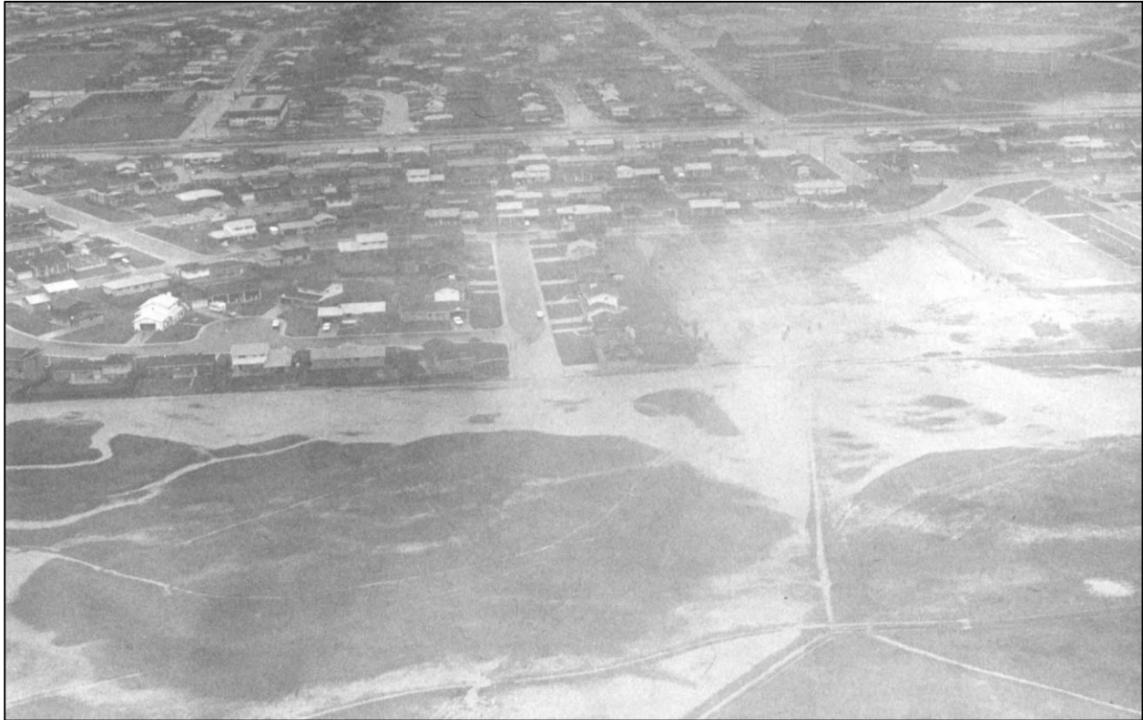
Figure 10- Dry Creek No. 2 Ditch at Kewanee Drive Looking West (1969)
