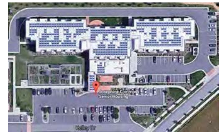
BCHA’s 70-unit Josephine Commons, showing large area required for parking.
