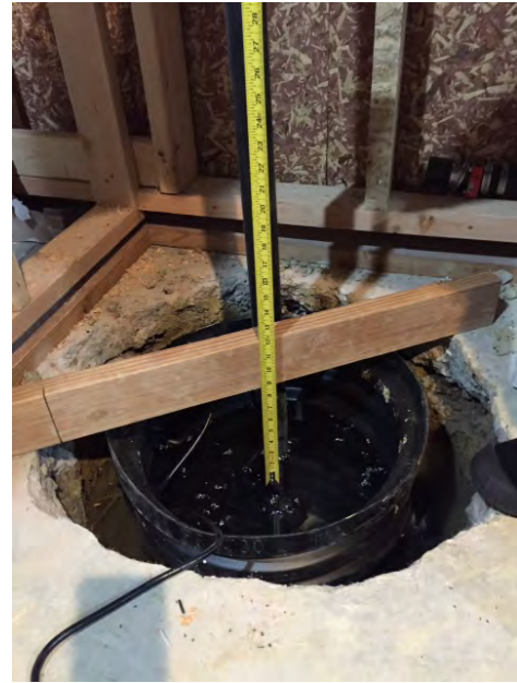
FIGURE 5 – RED FOX HILLS HIGH WATER TABLE A 9 INCHES BELOW THE TOP OF THE BASEMENT SLAB (TAKEN 11/9/2015)
