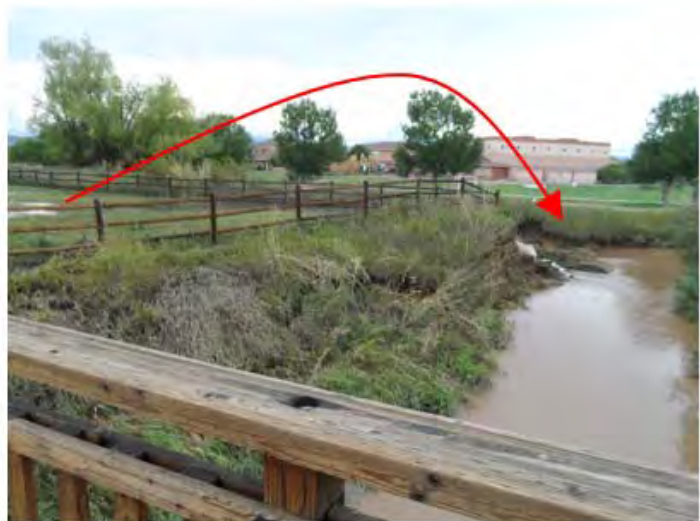
FIGURE 6 – DAVIS NO. 2, WESTERN TWIN LAKES DAM, OVERFLOWING DURING THE 2013 FLOODS. ARROW SHOWS PATH OF WATER FROM THE NE CORNER OF THE WESTERN DAM.
