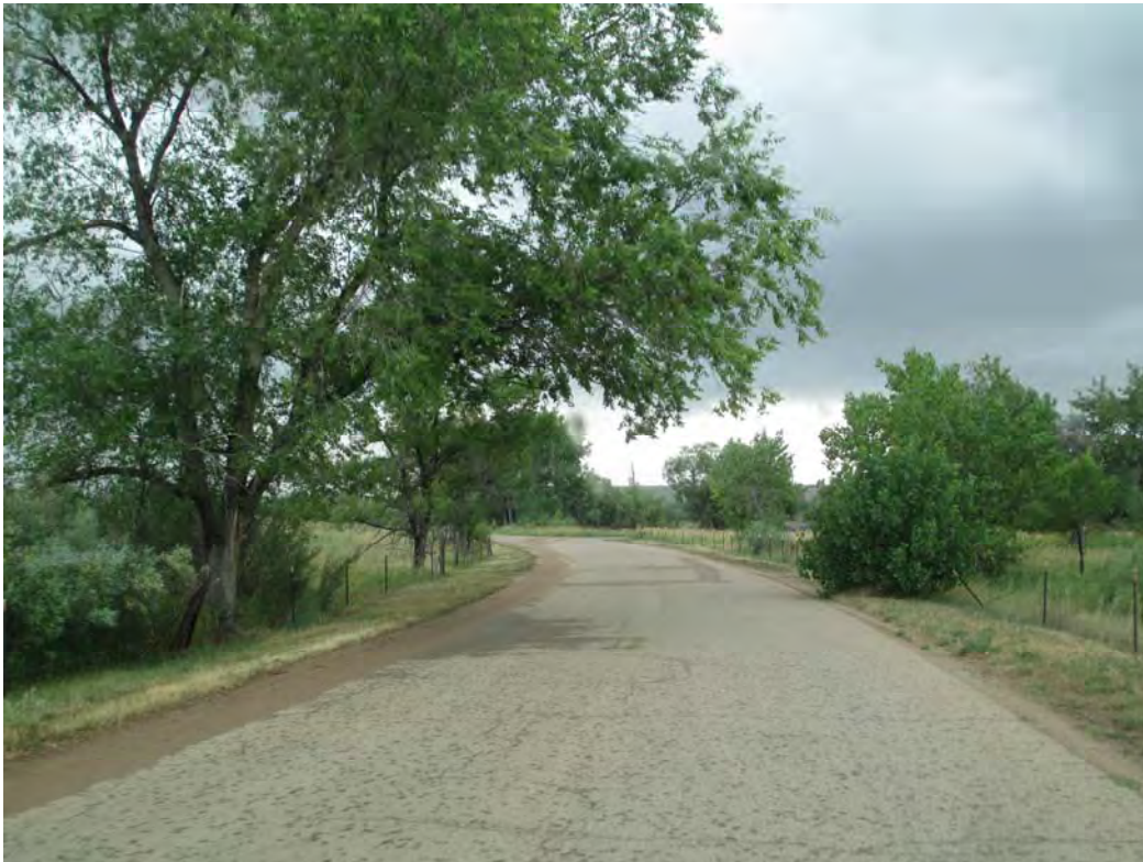
Photo 4 Loop Drive within CU South
