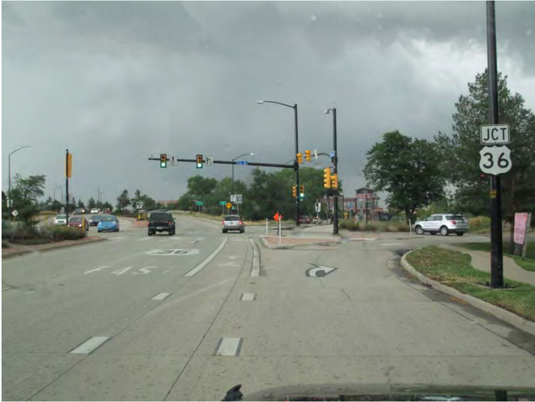
Photo 1 Eastbound Table Mesa Drive at Loop Drive
