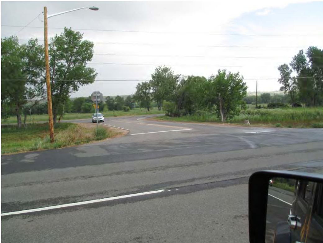
Photo 12 Marshall Road Connection to CO 93
