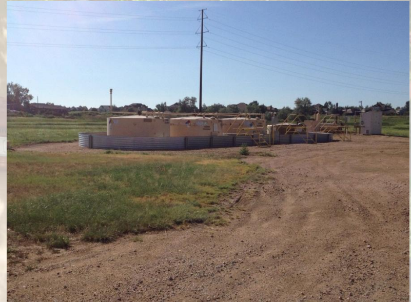
Similar tank battery w/containment no fencing (wellhead is just out of the picture on the right)
