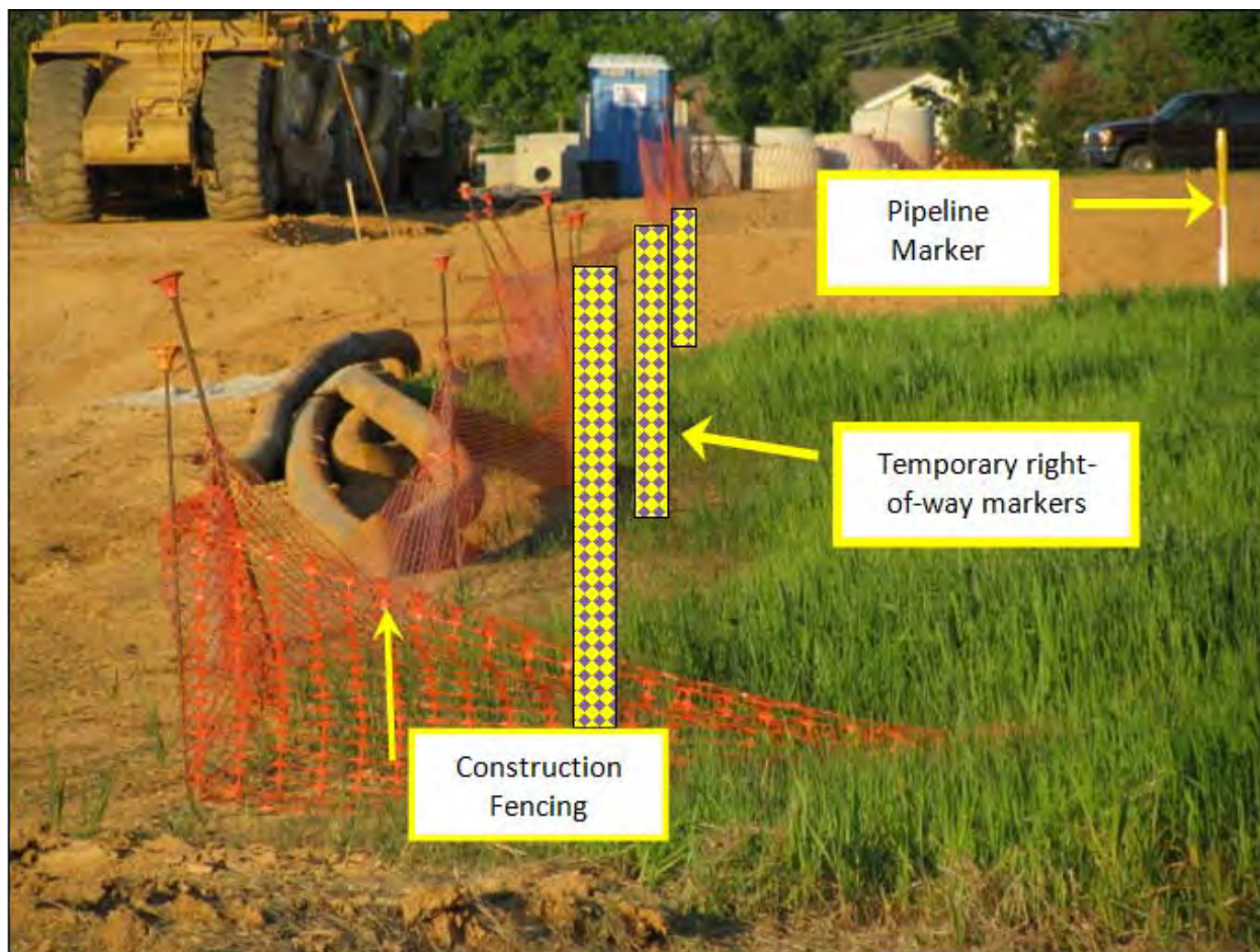
Construction site adjacent to transmission pipeline right-of-way – Example of use of temporary right-of-way markers and construction fencing – The markers along the left edge of the right-of-way are temporary right-of-way markers. The other marker is a transmission pipeline marker which indicates the location of the pipeline within the right-of-way. Notice the concrete pipe and heavy equipment located outside the right-of-way.
