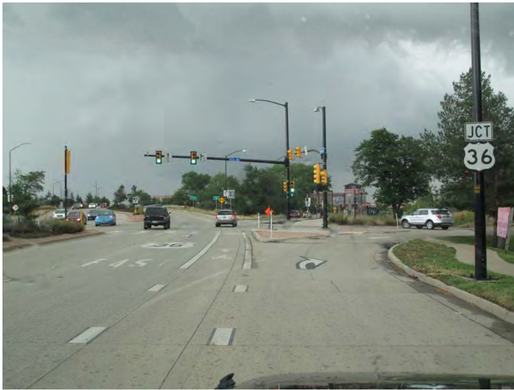
Photo 1 Eastbound Table Mesa Drive at Loop Drive
