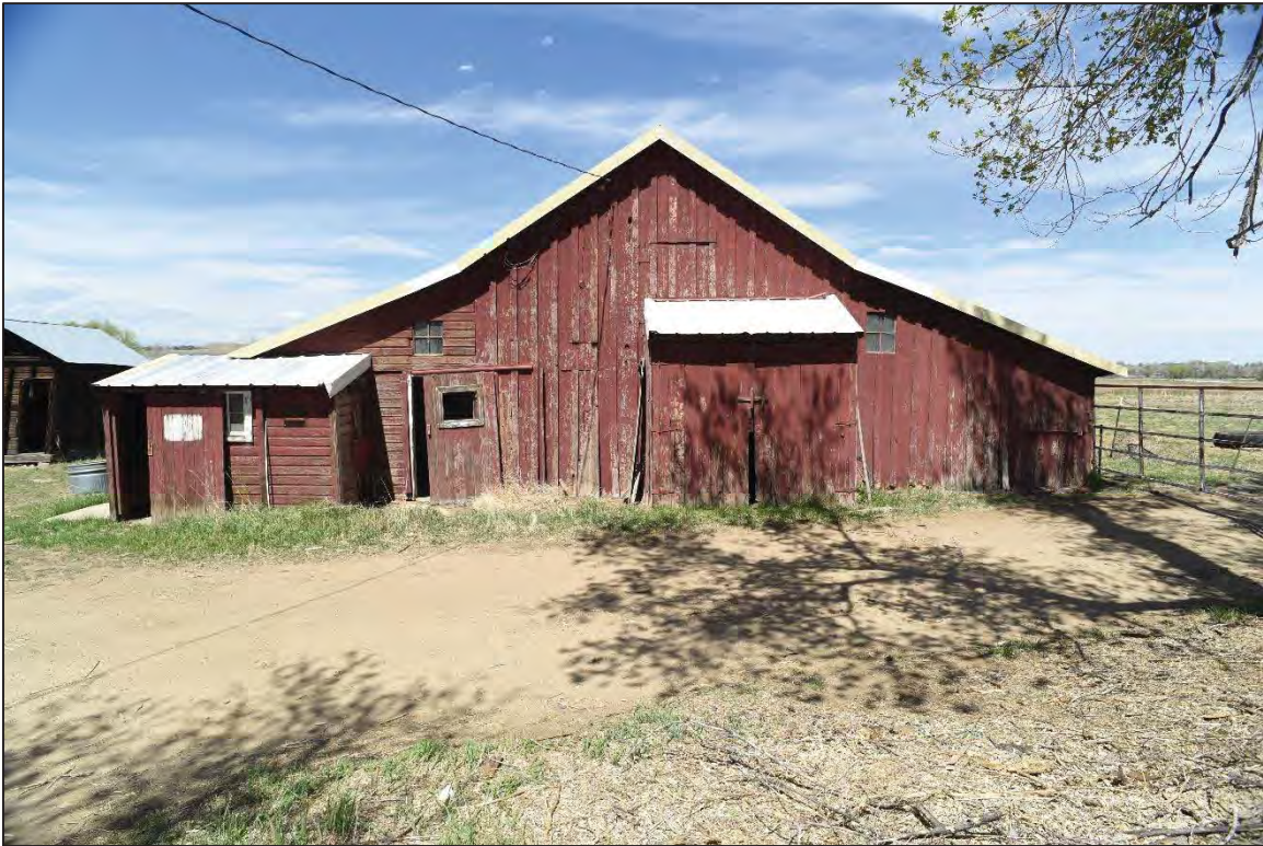
Photo 6212: Southern elevation of the Red Barn.
