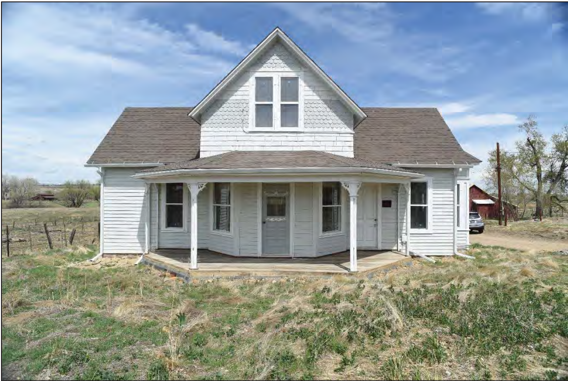
Photo 6166: Southern elevation of the Farm House.
