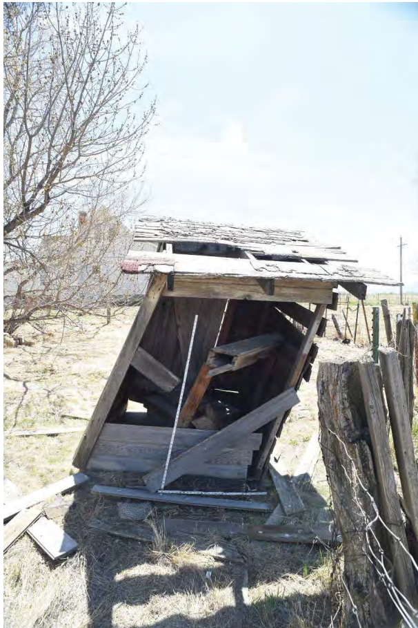
Photo 6217: Northern elevation of the outhouse.
