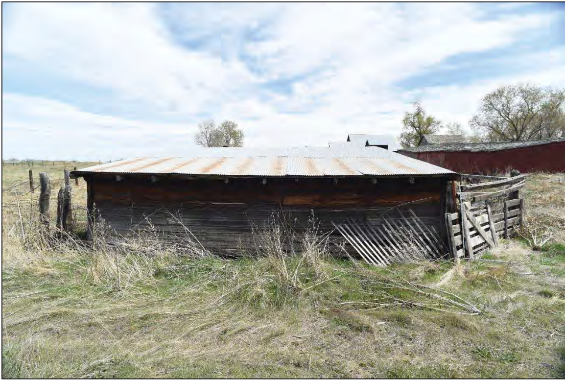
Photo 6185: Northern elevation of the Bull Shed.
