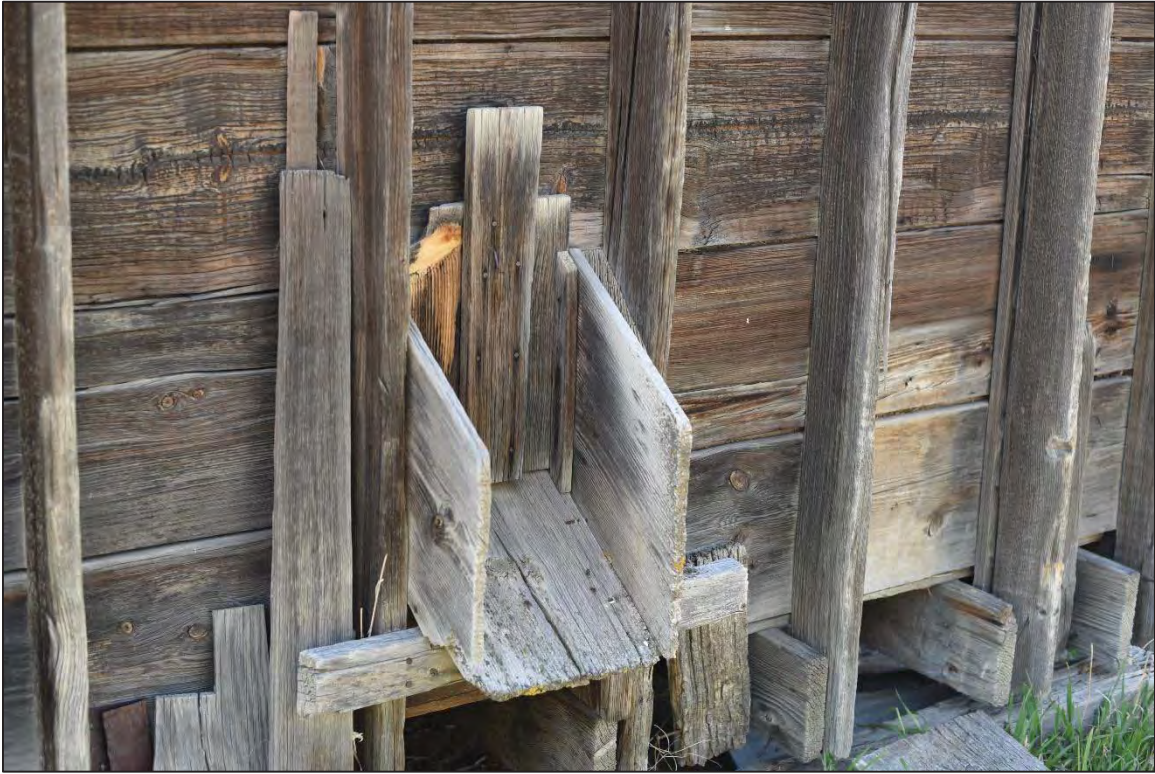
Photo 6227: Grain chute on western elevation of Chicken House.
