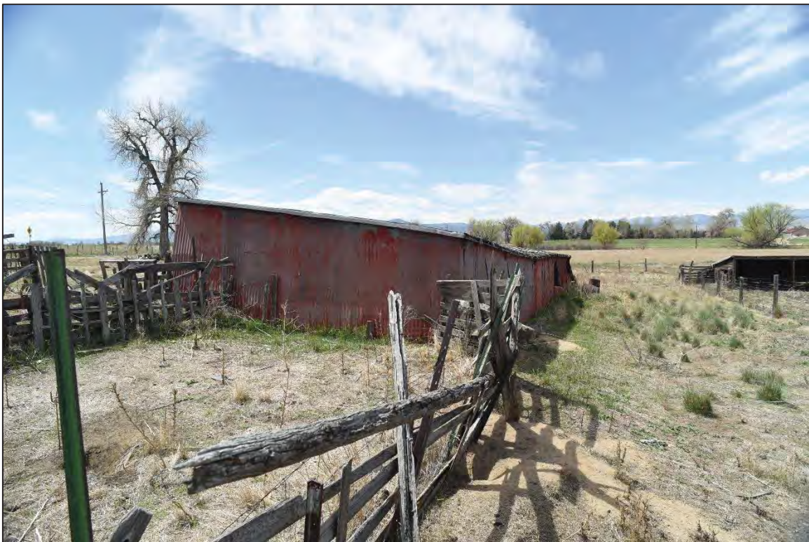
Photo 6189: Eastern elevation of the West Loafing Shed.
