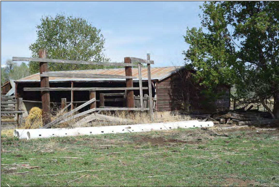
Photo 6391: Oblique view of southern and eastern elevations of Loafing Shed.
