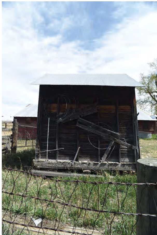
Photo 6196: Western elevation of the Corn Crib (inverted)
