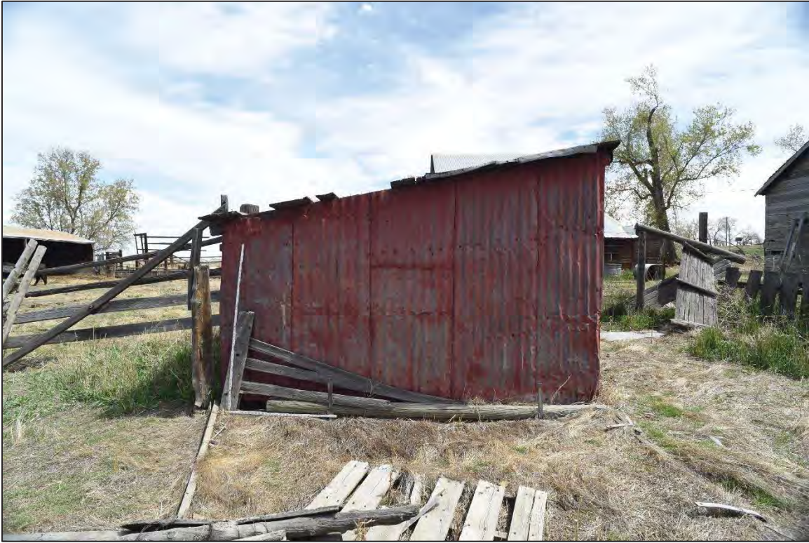
Photo 6190: Western elevation of the West Shed.
