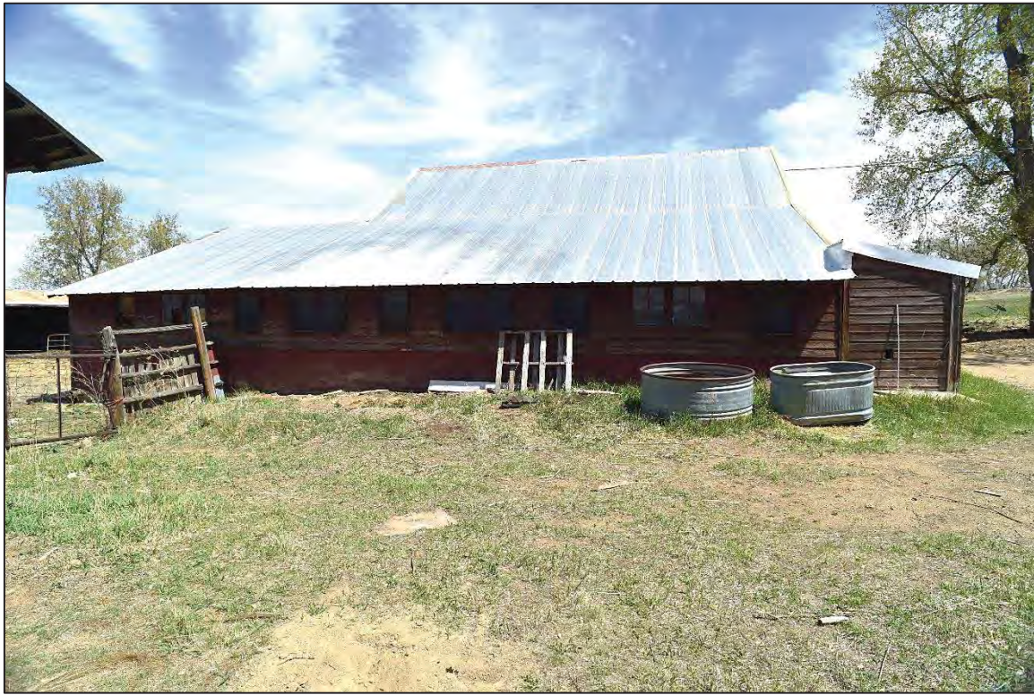
Photo 6211: Western elevation of the Red Barn.
