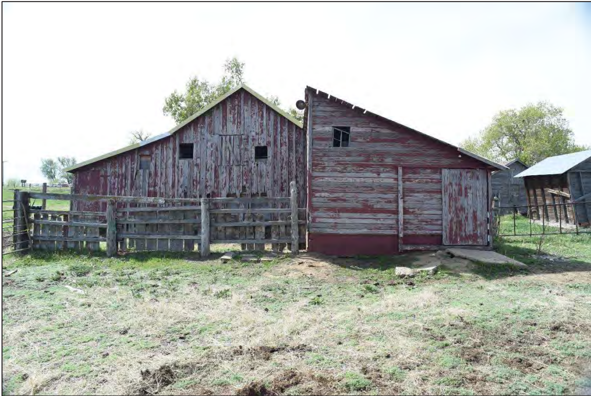
Photo 6412: Northern elevation of the Red Barn.
