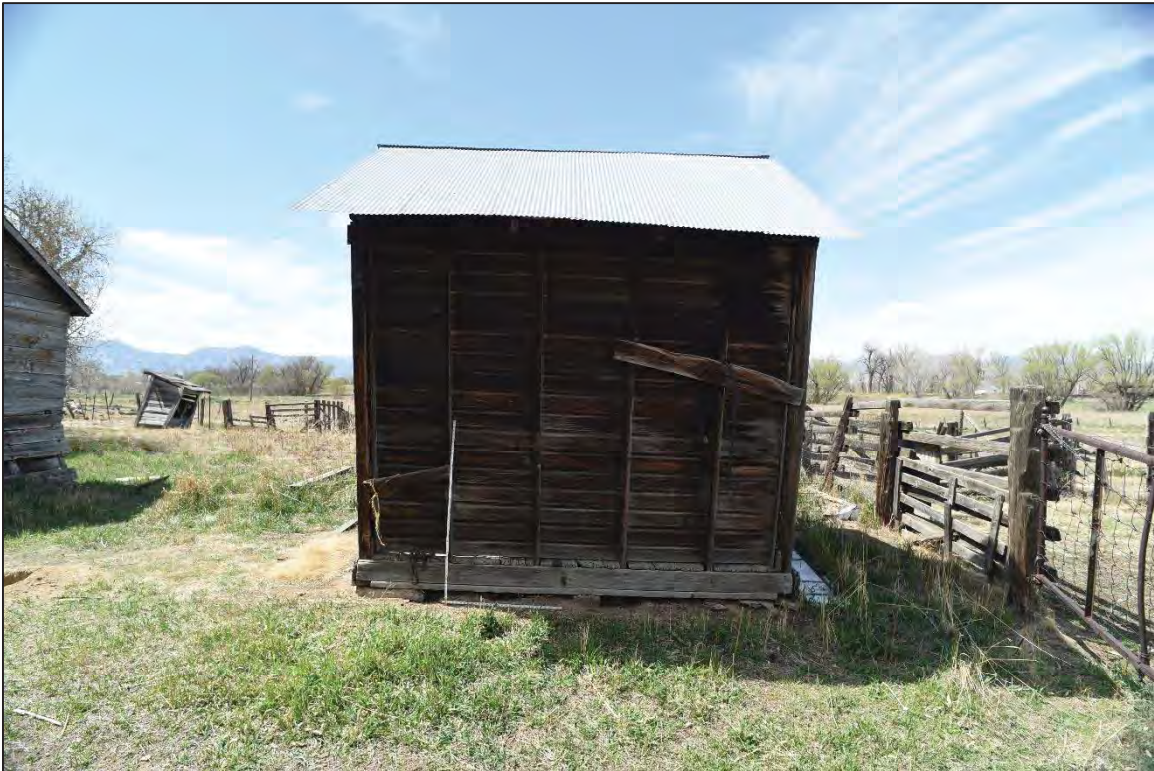
Photo 6200: Eastern elevation of the Corn Crib
