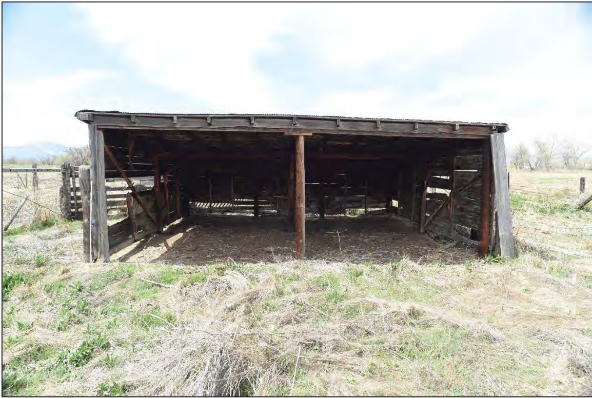
Photo 6181: Southern elevation of the Bull Shed.
