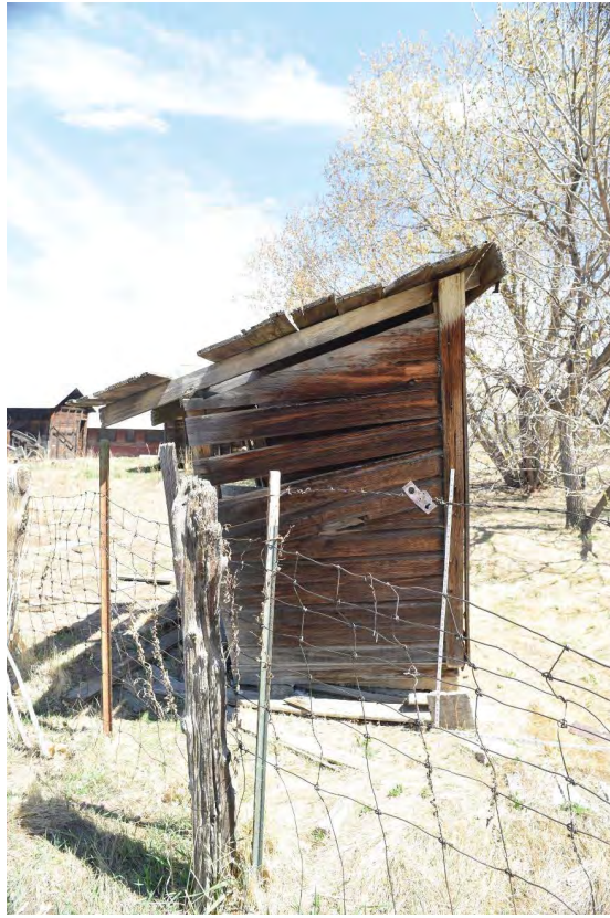
Photo 6216: Western elevation of the outhouse.
