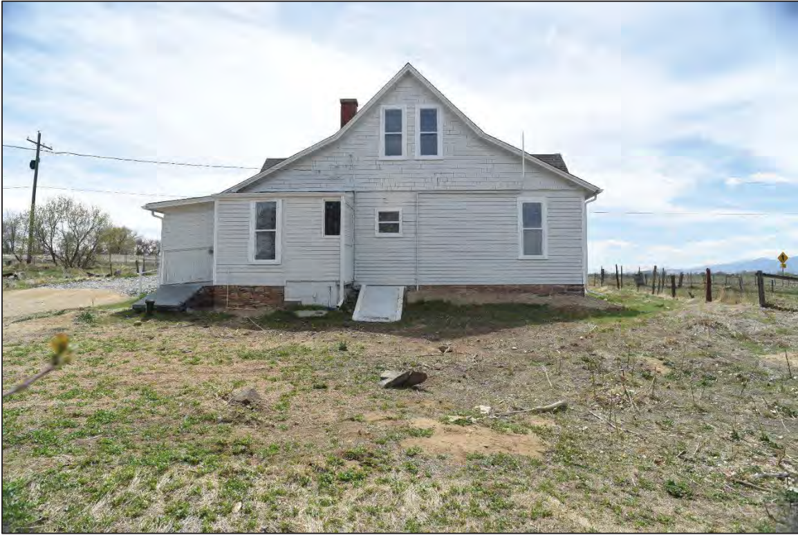
Photo 6174: Northern elevation of the Farm House.
