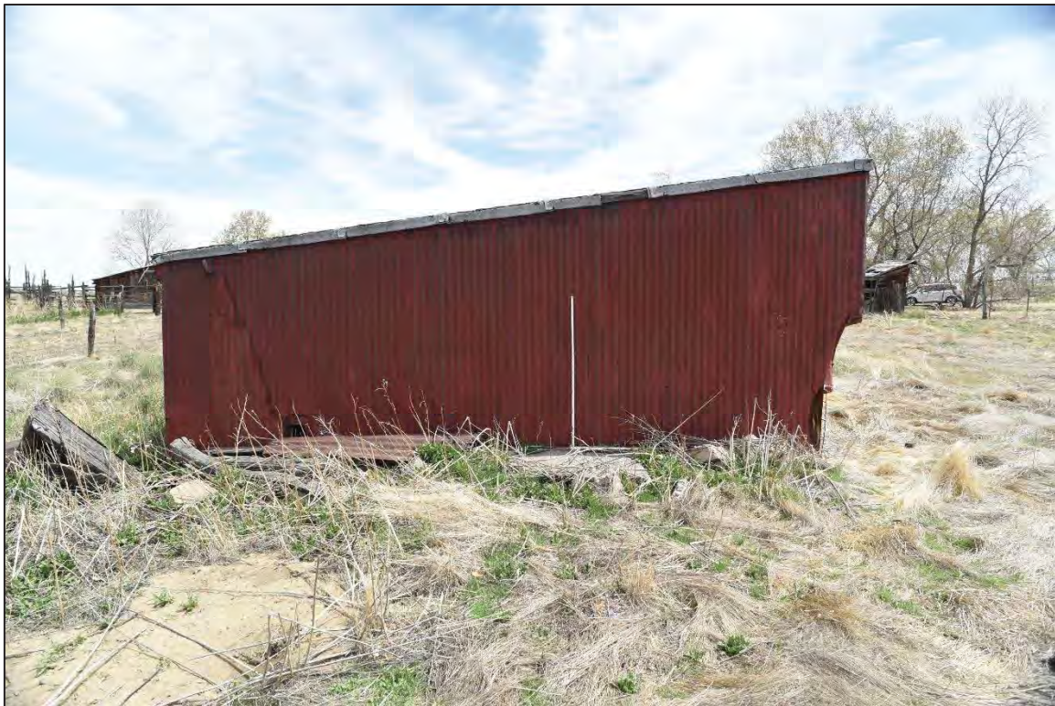
Photo 6179: Western elevation of the West Loafing Shed.
