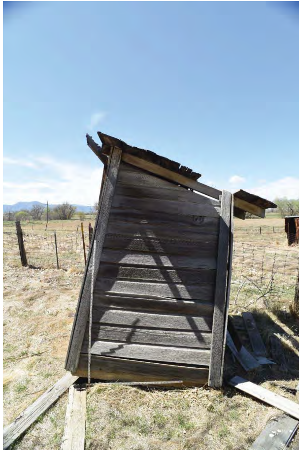
Photo 6214: Eastern elevation of the outhouse.
