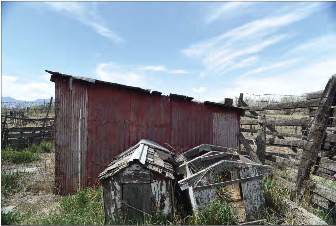
Photo 6195: Eastern elevation of the West Shed.
