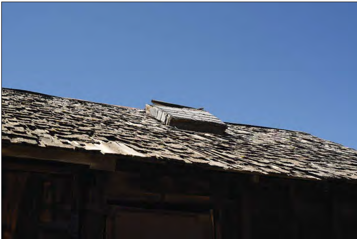
Photo 6228: Hatch on east-facing roof pitch of Chicken House.
