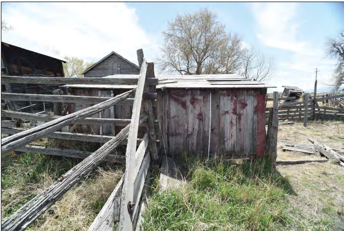
Photo 6192: Northern elevation of the West Shed.
