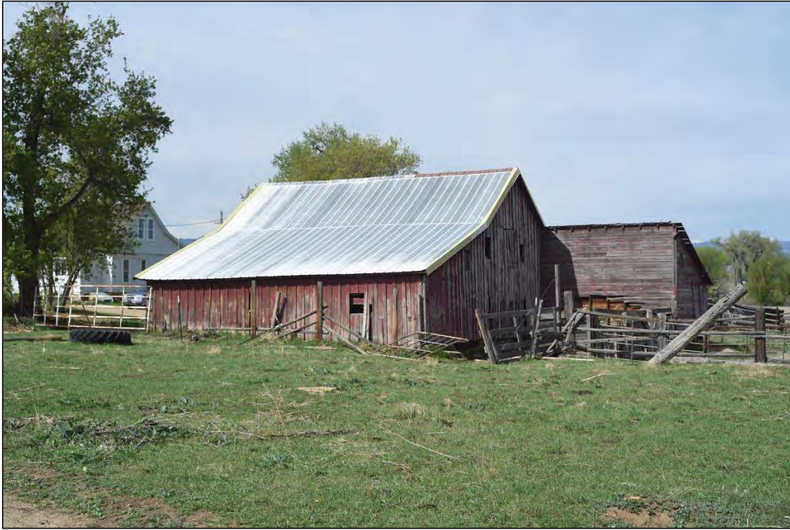
Photo 6384: Oblique view of eastern and northern elevations of the Red Barn.
