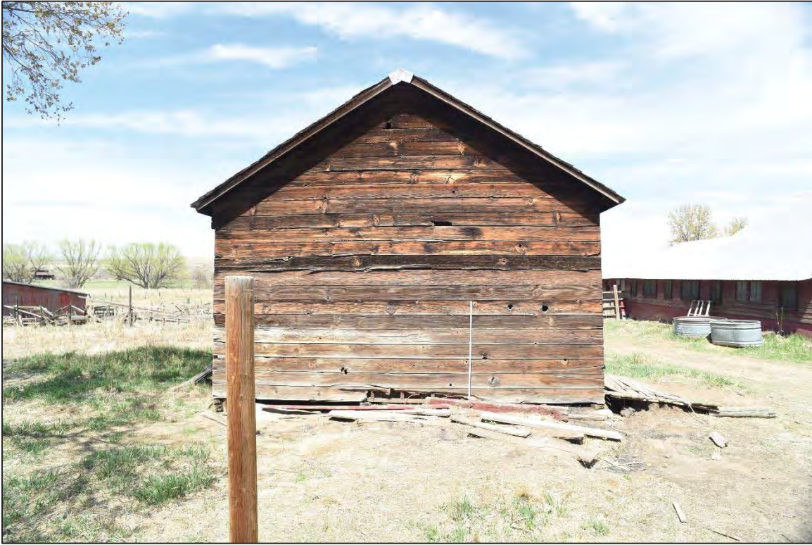
Photo 6207: Southern elevation of the Chicken House.
