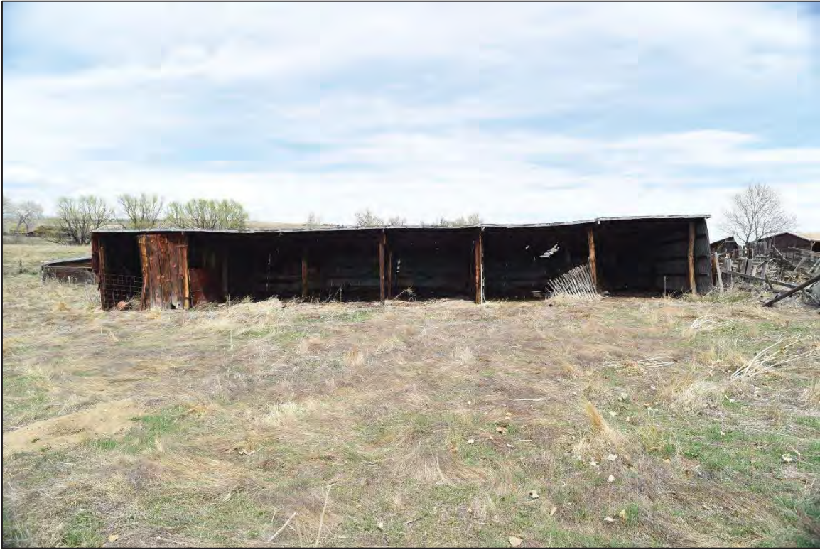
Photo 6177: Southern elevation of West Loafing Shed.
