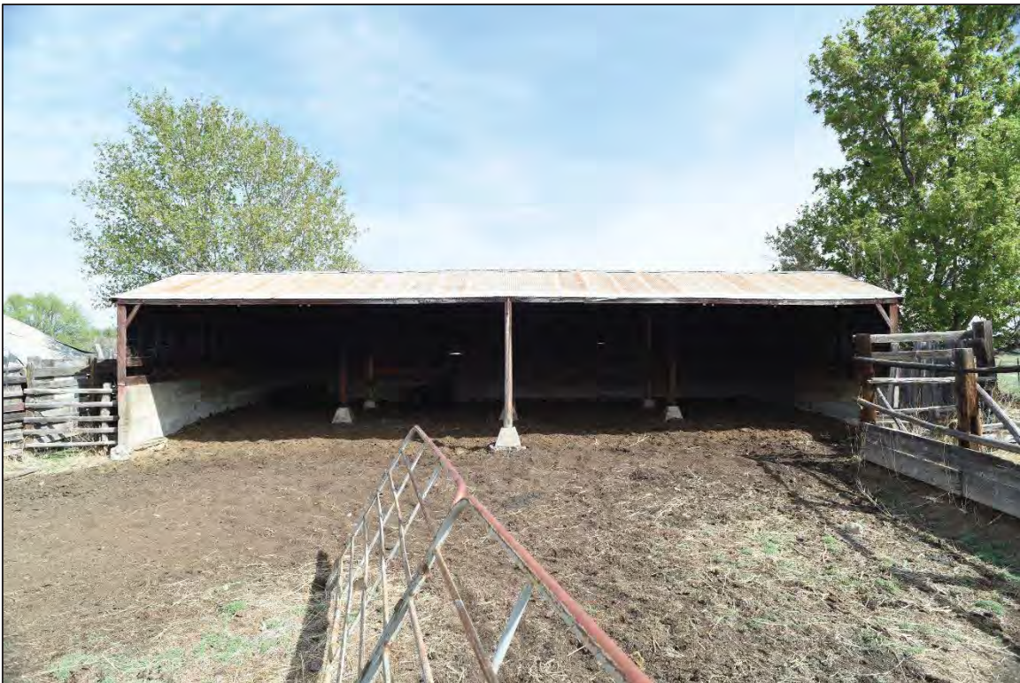
Photo 6407: Southern elevation of main Loafing Shed section.
