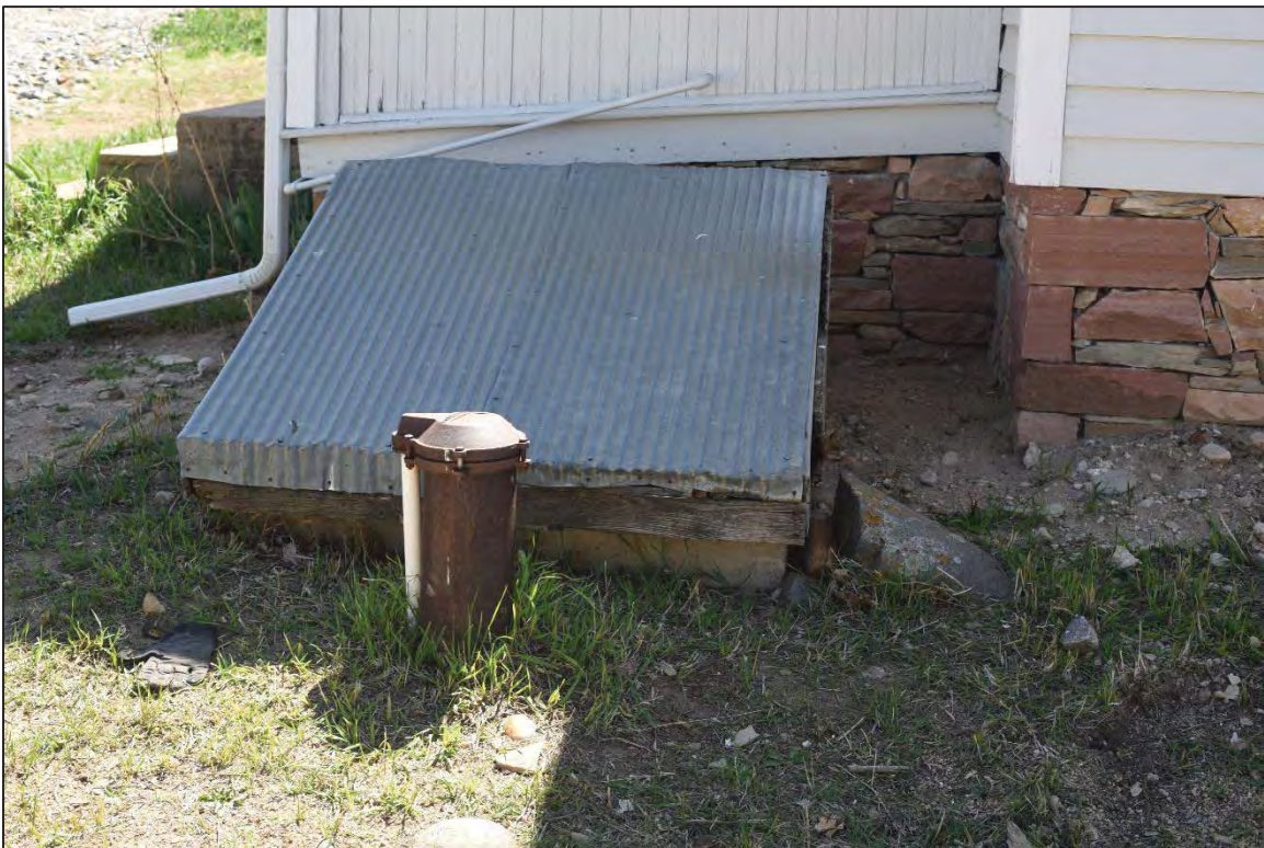
Photo 6230: Well head at northeast corner of Farm House.
