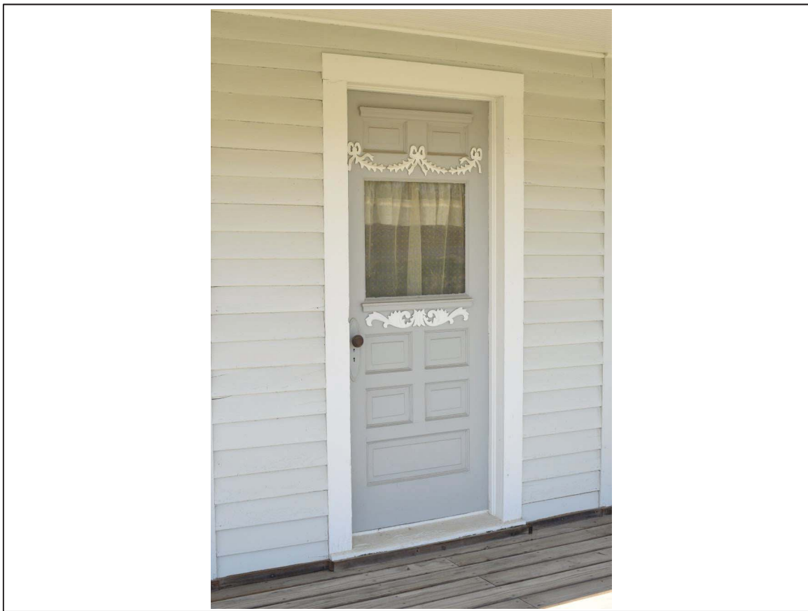
Photo 6237: Ornamental door (primary entry door) with carved wood appliques on southern elevation of Farm House on covered porch.
