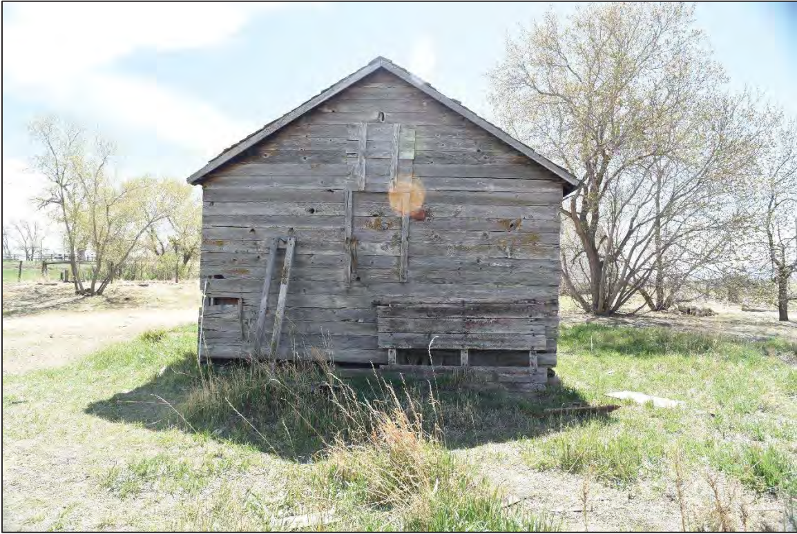
Photo 6203: Northern elevation of the Chicken House.
