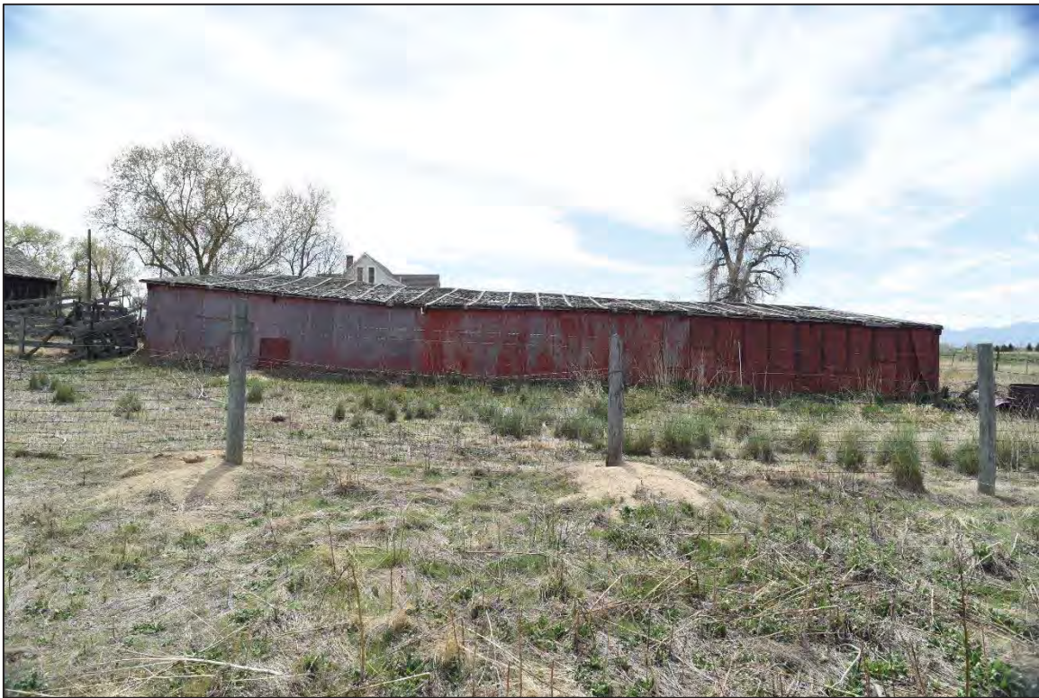
Photo: 6180: Northern elevation of the West Loafing Shed.
