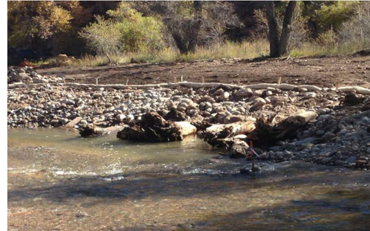
Downstream view: Type 2 large woody structure at main channel St. 89+90 right bank .
