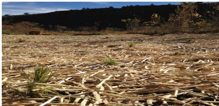
Downstream View: Wood straw mulch installed in overflow channel D
