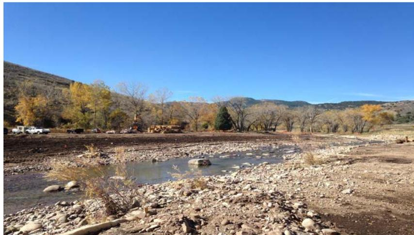
Upstream View: Completed fine grading of main channel between St. 76+00 to 82+50 and soil conditioned floodplain.
