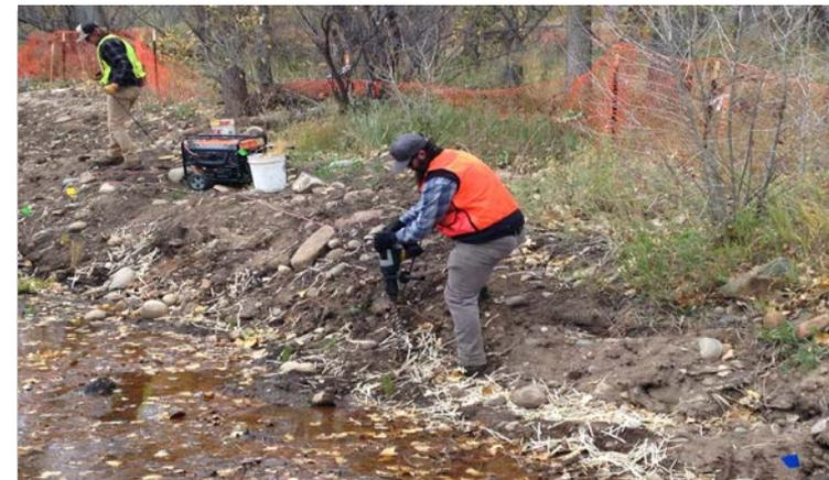
Upstream View, left bank: Hammer drilling to install perennial tubelings in overflow channel E
