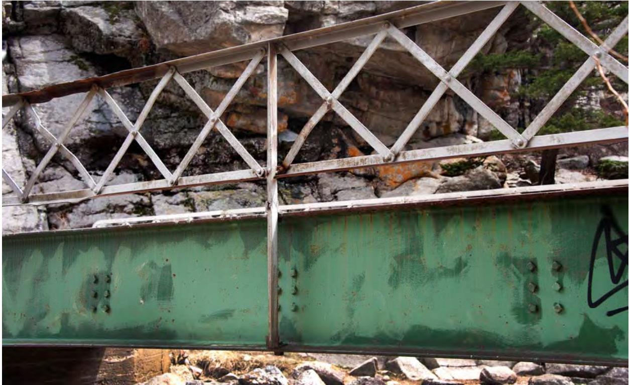
Upper Castle Rock Bridge, detail of west girder, showing lattice guardrail and bolts connecting transverse joists to girder. View to northeast.
