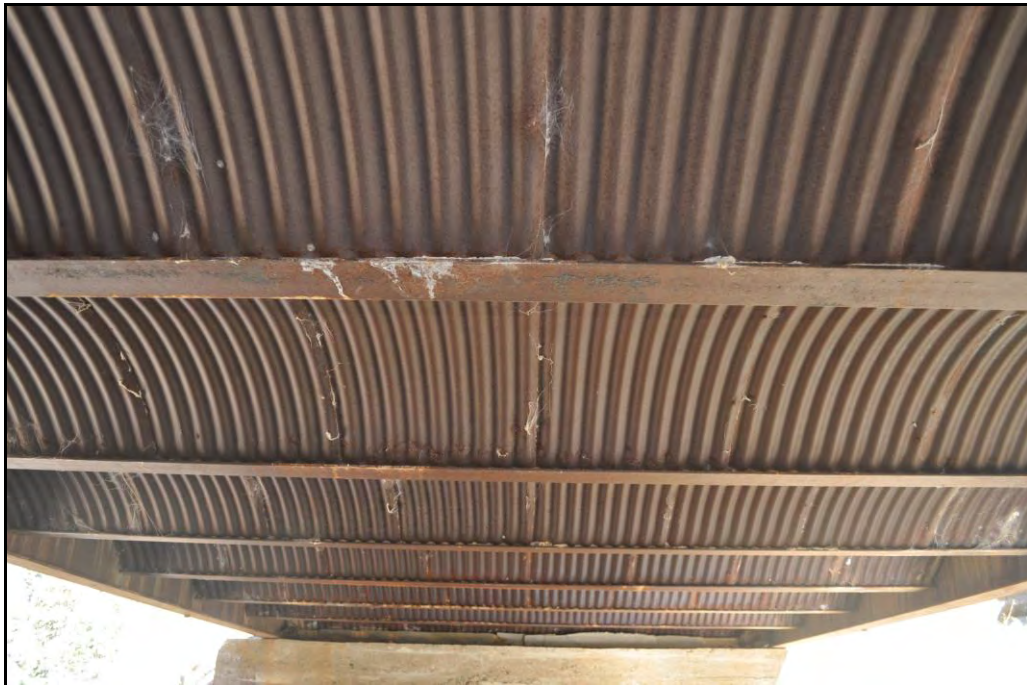
View showing I-beams, I-beam joists and corrugated steel culvert sections
