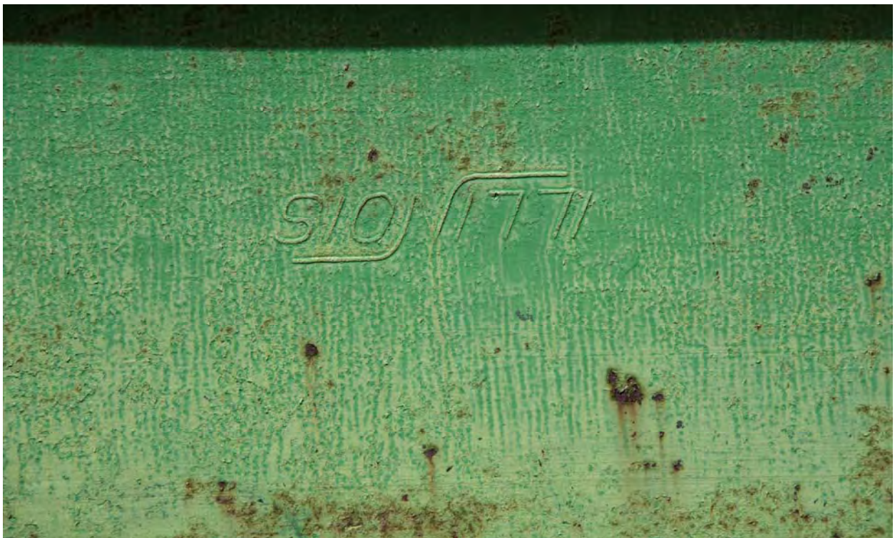
Upper Castle Rock Bridge, detail of girder, showing steel manufacturer's mark. View to east.
