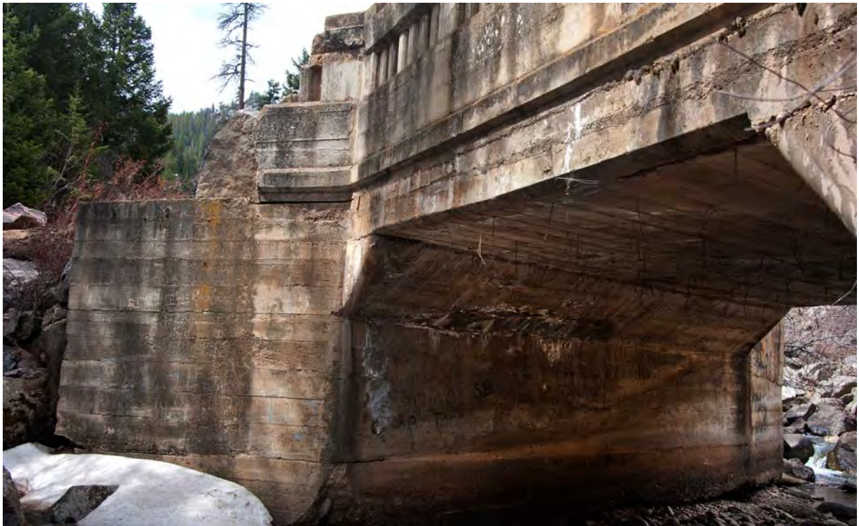
Lower Castle Rock Bridge, south abutment, showing guardrail damage in southeast corner. View to west.
