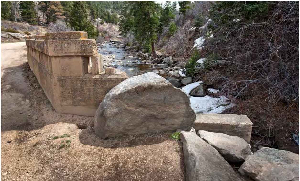
Lower Castle Rock Bridge, east-side guardrail, showing damage in southeast corner. View to northeast.
