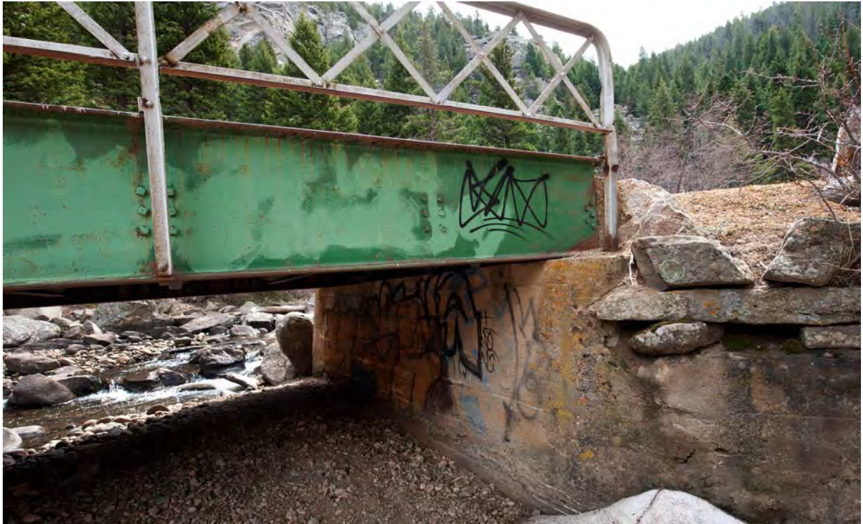
Upper Castle Rock Bridge, south abutment, showing bearing of west girder. View to southeast.
