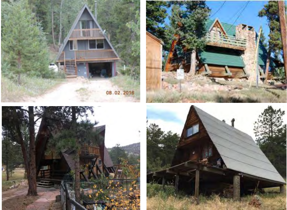
Figures 85 through 88. Clockwise from upper left: Elevated A-frame and enclosed foundation (91 Doe Trail, Nederland); exposed rafter tails resting on knee wall (98 Mine Lane, Unincorporated); Exposed rafter tails extending to the ground (208 Wild Tiger, Unincorporated); Concrete pier foundation (1120 Lewis Lane, Unincorporated). 195
