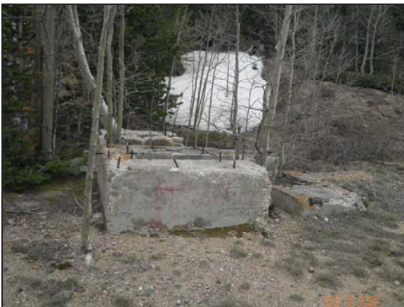
Foundations at unidentified site
