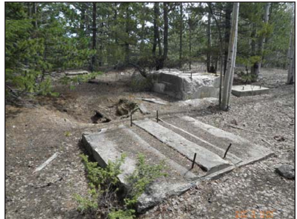
Foundations at unidentified site
