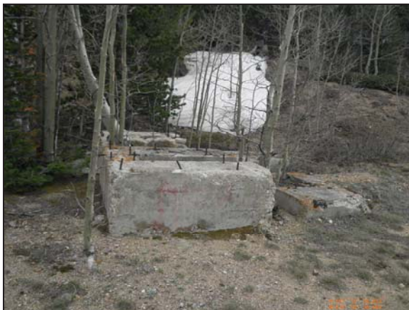
Foundations at unidentified site
