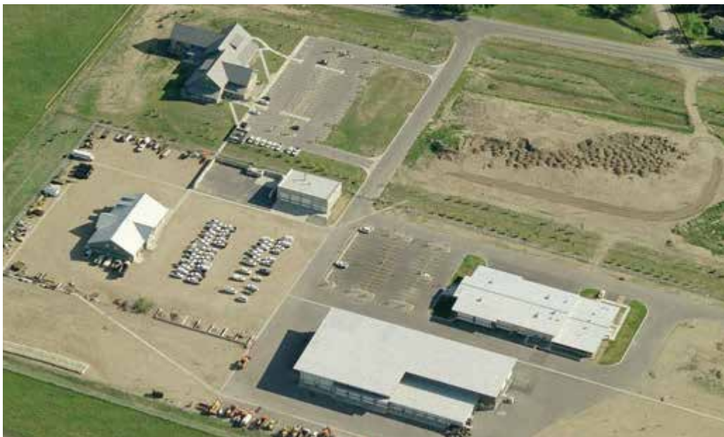
Parks & Open Space and Transportation Campus, in Longmont aerial view. Circa 2007.
