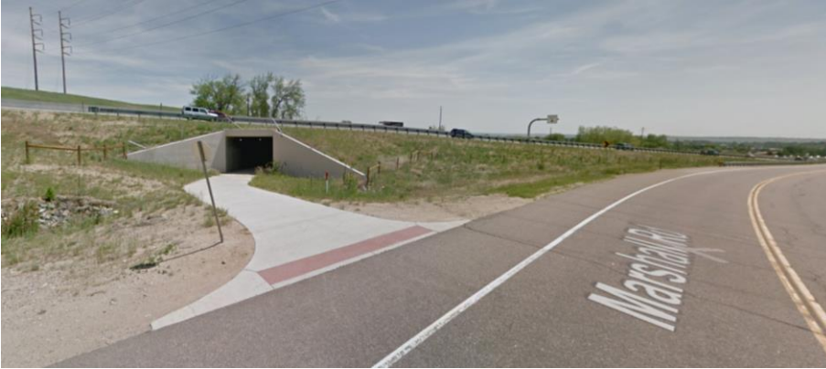
Bicycle and Pedestrian Underpass providing a connection from SH 170 Marshall Dr to the US 36 Bikeway under US 36
