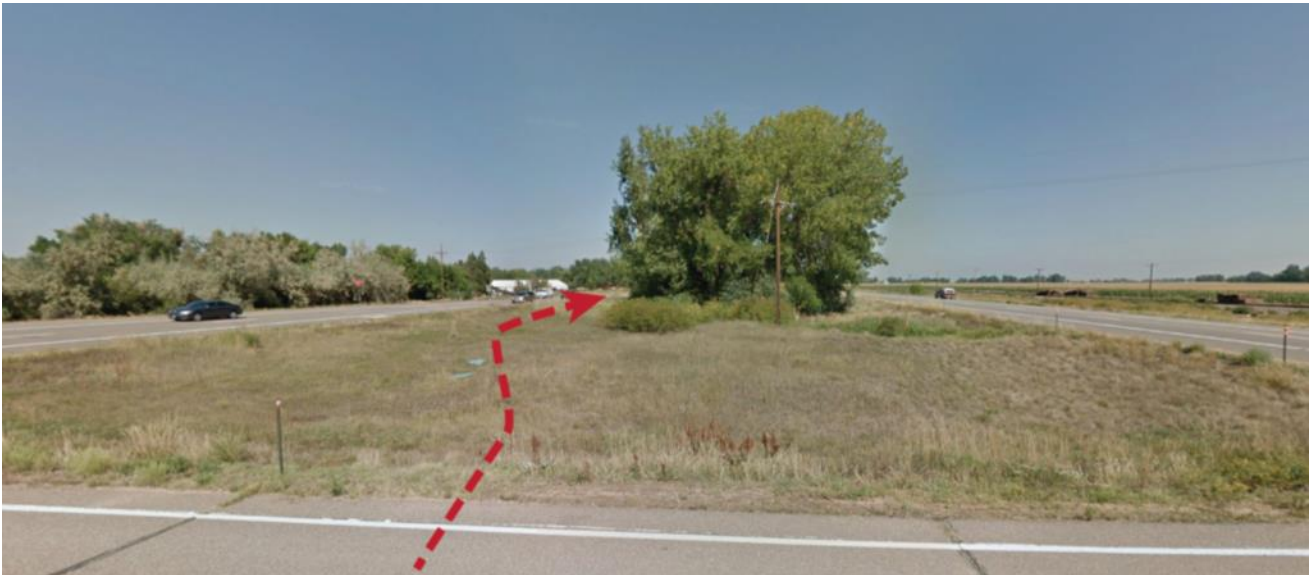
Current “poor” pavement condition of the SH 119 Bikeway. Source: Google Streetview
