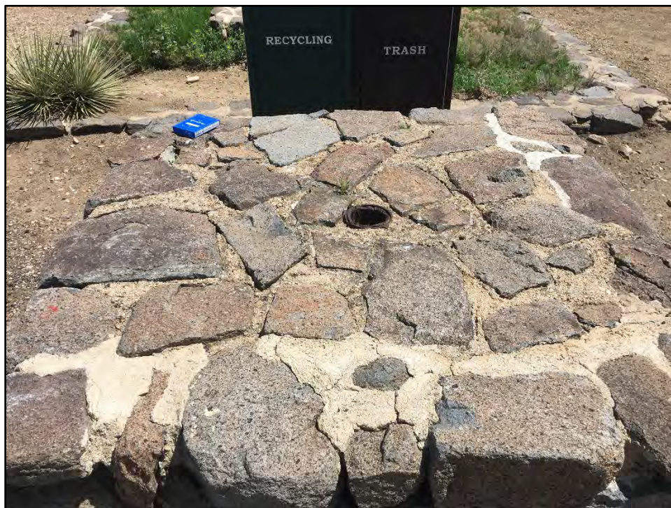
Detail view showing top of north flag pole pedestal with centered pipe hole that previously held the flagpole. June 4, 2019
