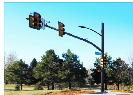
Figure 9: Acceptable Small Cell Design on a Traffic Pole
