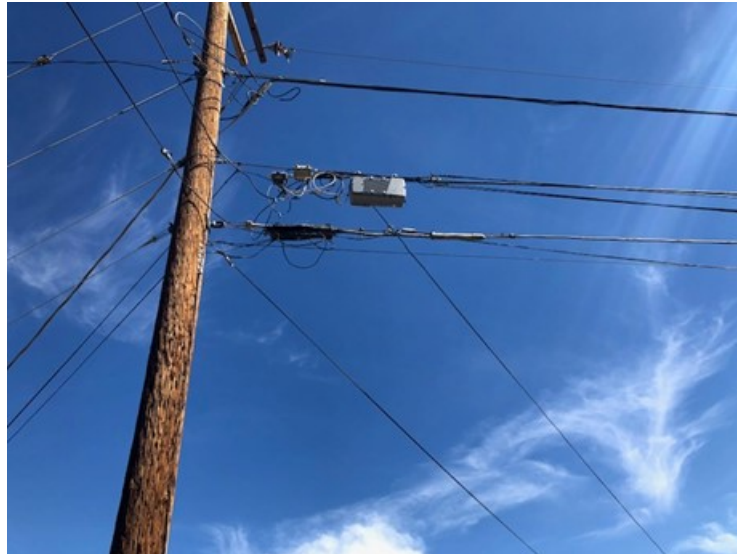
Figure 18 An example of a strand mountable eNodeB
