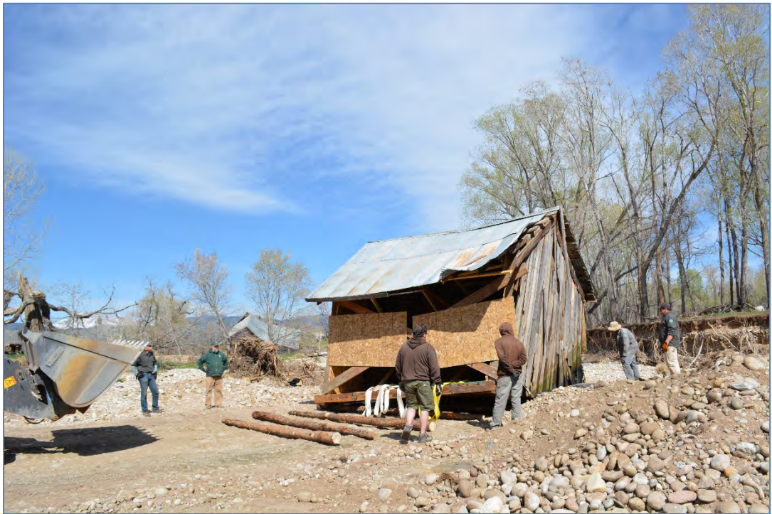
Parks and Open Space Buildings and Historic Preservation work group moving granary. Note the logs on the ground in front of the granary that allowed the building to be rolled to temporary location while being pulled by front end loader. View to the northwest. April 24, 2014
