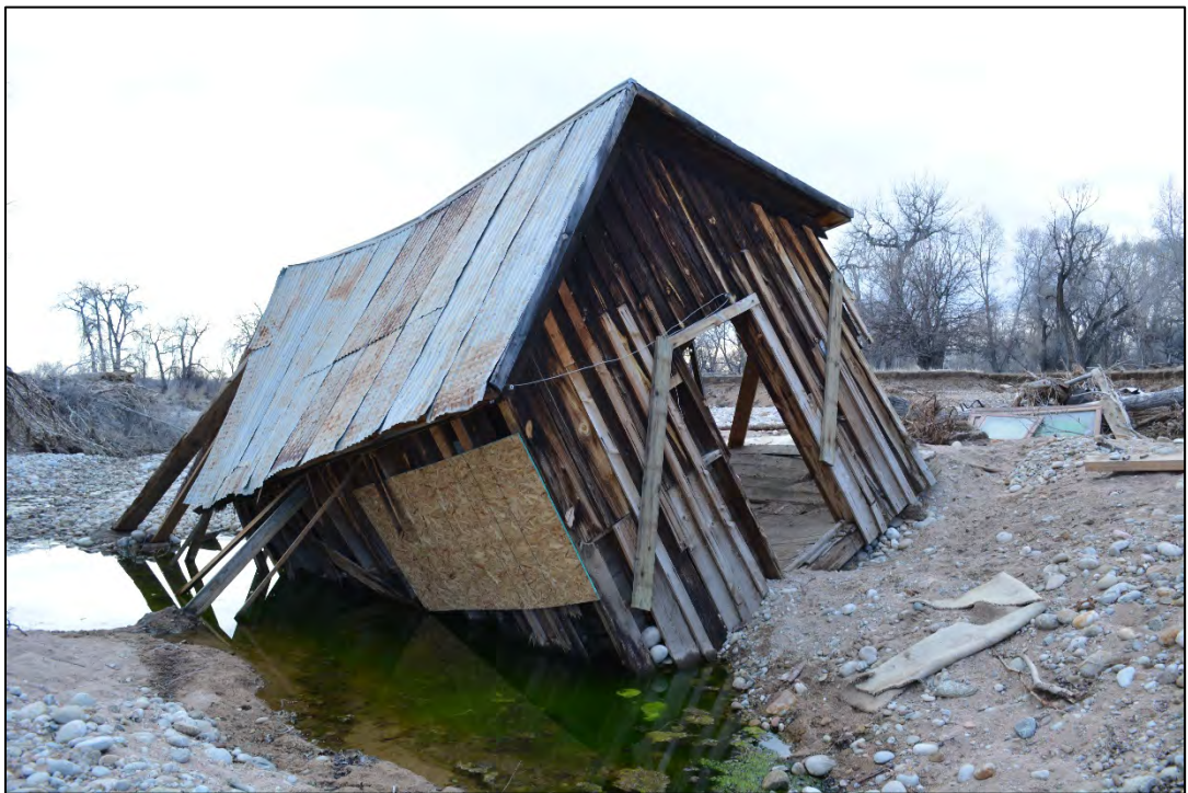
Granary location in large flood scour area showing temporary stabilization. View to the east. March 26, 2014
