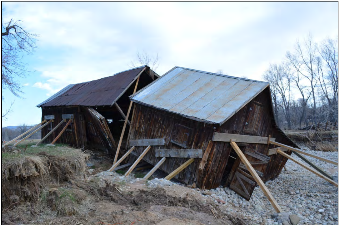
Southeast barn damage detail showing temporary stabilization March 26, 2014
