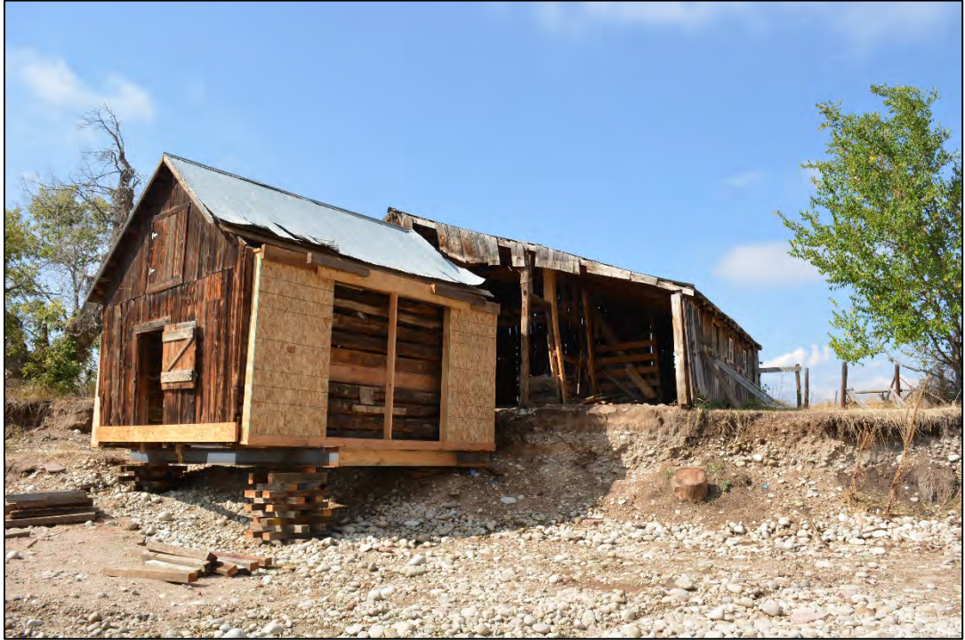
Eastern barn section prepped to be lifted. View to the southwest. October 5, 2015
