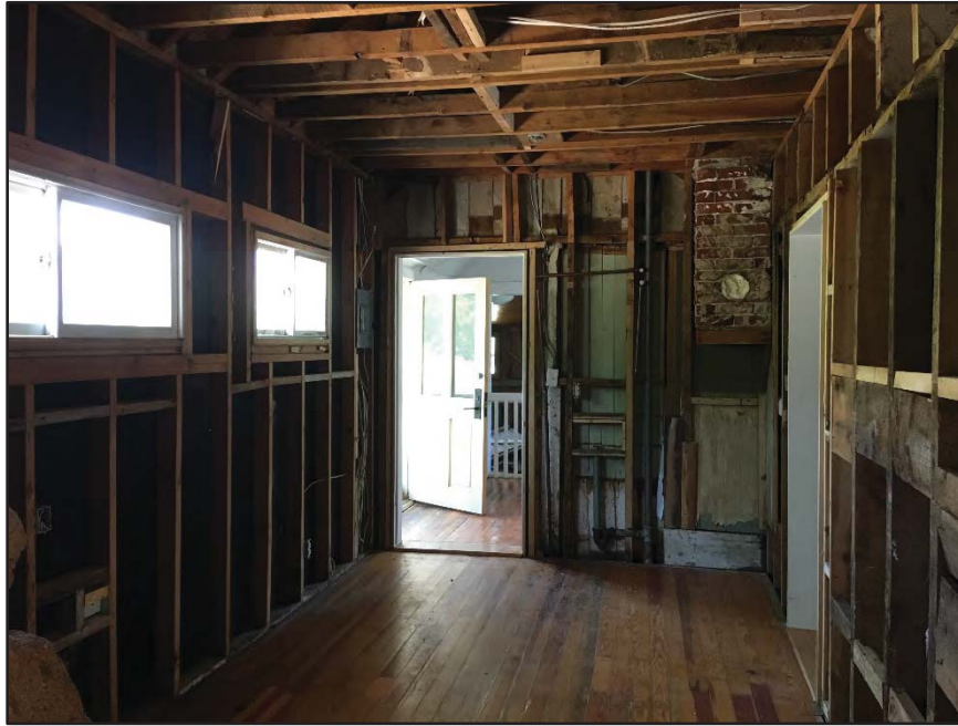
Tumbleson House – interior rear addition looking east
