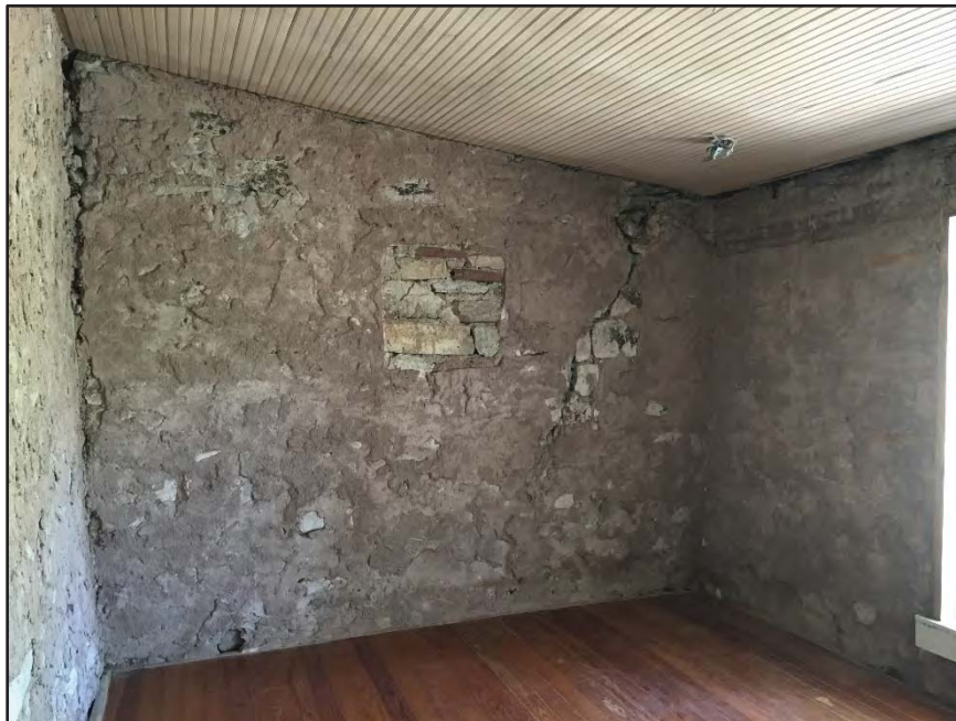
Tumbleson House – interior southwest elevation detail
