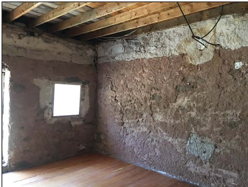
Tumbleson House – interior southwest elevation detail
