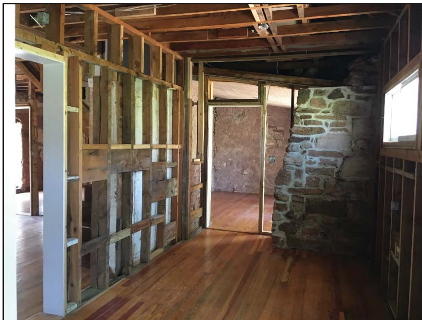
Tumbleson House – interior rear addition looking west
