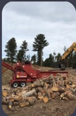
Grinding woody biomass at the Nederland CFSY.
