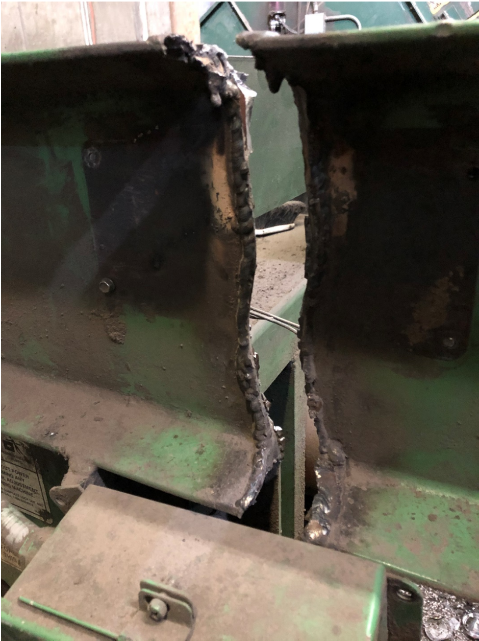
Opposite side view of top rail Channel steel
