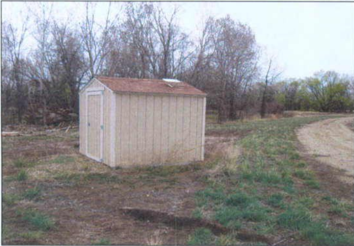
1. Pump house on east side of clay-lined pond.
