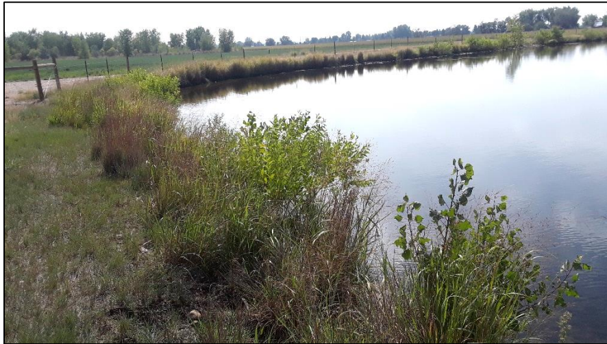
Photo 35. View of northeastern shoreline of pond 7 in area south of river. Pond slopes are at 3H:1V or flatter with good vegetative cover.
