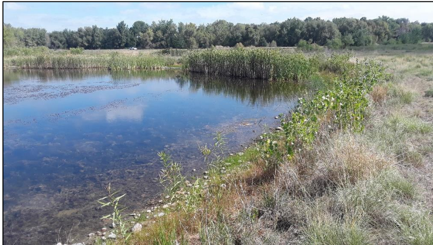
Photo 20. View of eastern shoreline of pond 3 in area south of river. Pond slopes are at 3H:1V or flatter with good vegetative cover.
