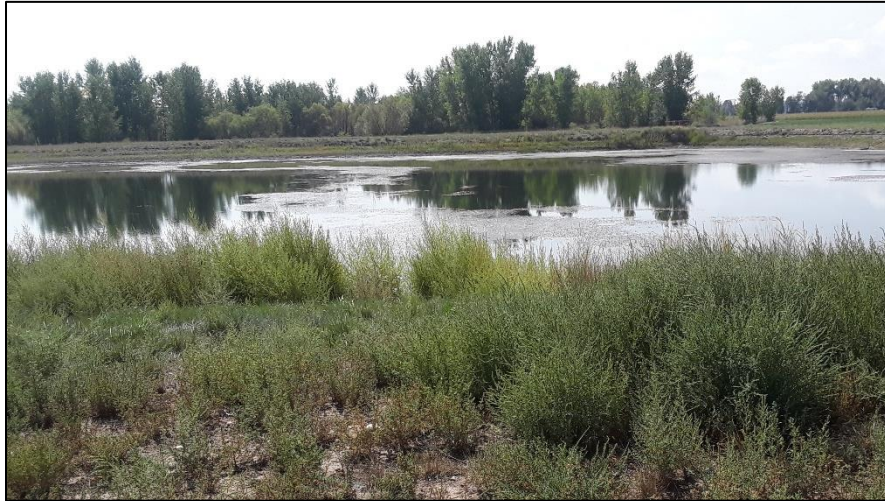
Photo 28. View of southern shoreline of pond 5 in area south of river. Pond slopes are at 3H:1V or flatter with good vegetative cover. Kochia covers much of grasses along northern shoreline (foreground).
