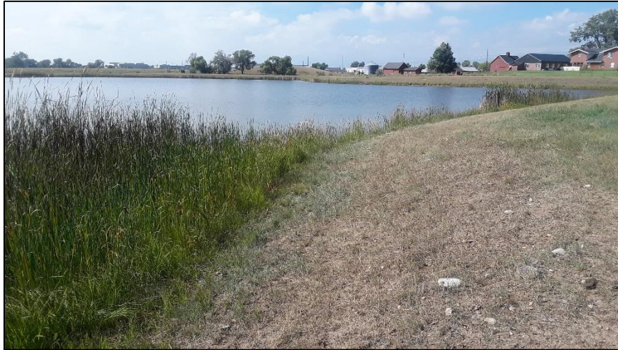
Photo 19. View of northern shoreline of pond 2 in area south of river. Pond slopes are at 3H:1V or flatter with good vegetative cover.
