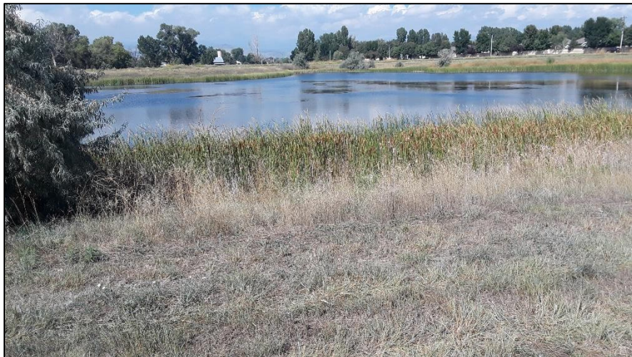
Photo 3. View of eastern shoreline of west pond in area north of river. Pond slopes are at 3H:1V or flatter with good vegetative cover.
