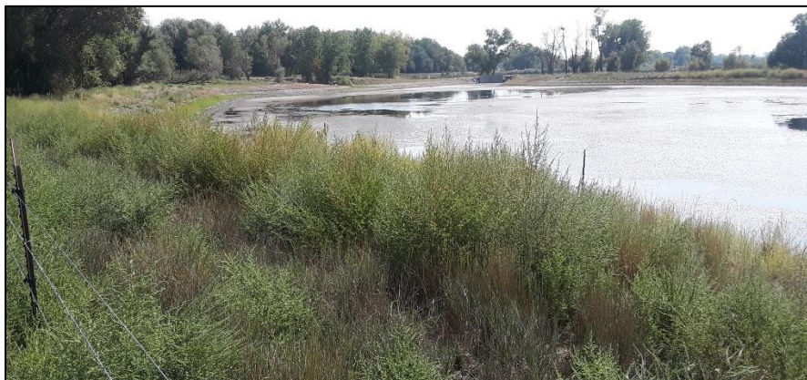
Photo 33. View of northwestern shoreline of pond 6 in area south of river. Pond slopes are at 3H:1V or flatter with good vegetative cover (Kochia covering much of grasses along this section).
