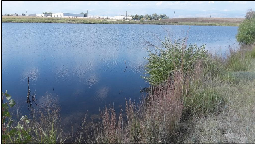
Photo 37. View of northern shoreline of pond 7 in area south of river. Pond slopes are at 3H:1V or flatter with good vegetative cover.
