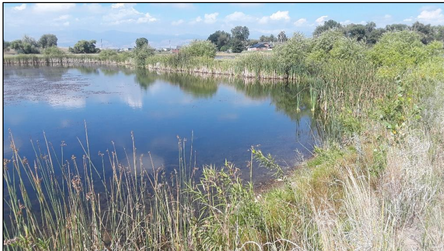
Photo 38. View of northwestern shoreline of pond 7 in area south of river. Pond slopes are at 3H:1V or flatter with good vegetative cover.
