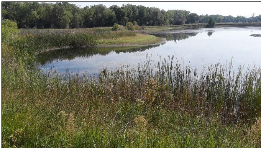
Photo 23. View of northwestern shoreline of pond 4 in area south of river. Pond slopes are at 3H:1V or flatter with good vegetative cover.
