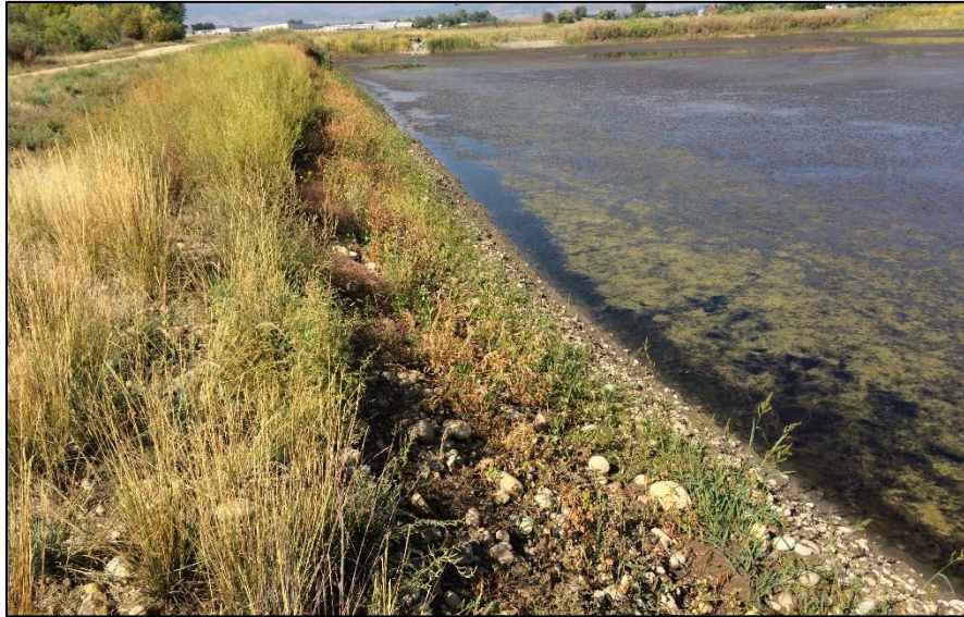
Photo 31. View of southern shoreline of pond 6 in area south of river. Pond slopes are at 3H:1V or flatter with good vegetative cover.
