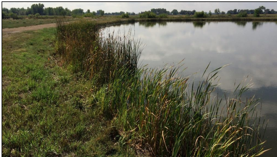
Photo 18. View of eastern shoreline of pond 2 in area south of river. Pond slopes are at 3H:1V or flatter with good vegetative cover.
