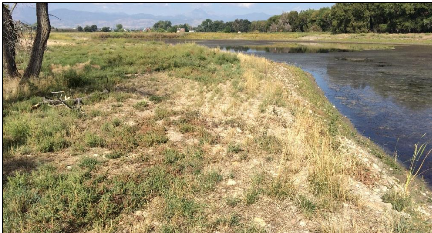
Photo 30. View of southeastern shoreline of pond 6 in area south of river. Pond slopes are at 3H:1V or flatter with good vegetative cover.
