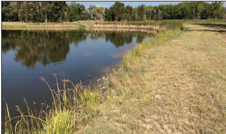
Photo 17. View of northeastern shoreline of pond 2 in area south of river. Pond slopes are at 3H:1V or flatter with good vegetative cover.
