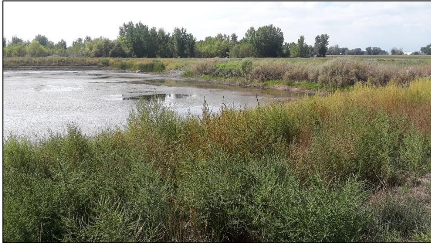
Photo 34. View of western shoreline of pond 6 in area south of river. Pond slopes are at 3H:1V or flatter with good vegetative cover (Kochia covering much of grasses along this section).
