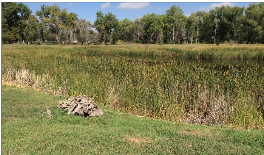
Photo 15. View of southern shoreline of pond 1 in area south of river. Pond slopes are at 3H:1V or flatter with good vegetative cover.
