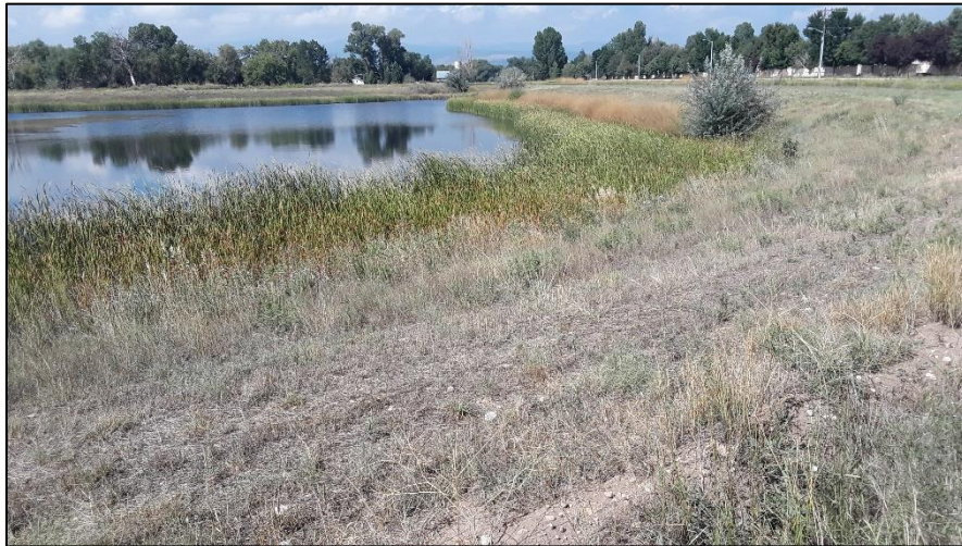
Photo 2. View of northeastern shoreline of west pond in area north of river. Pond slopes are at 3H:1V or flatter with good vegetative cover.
