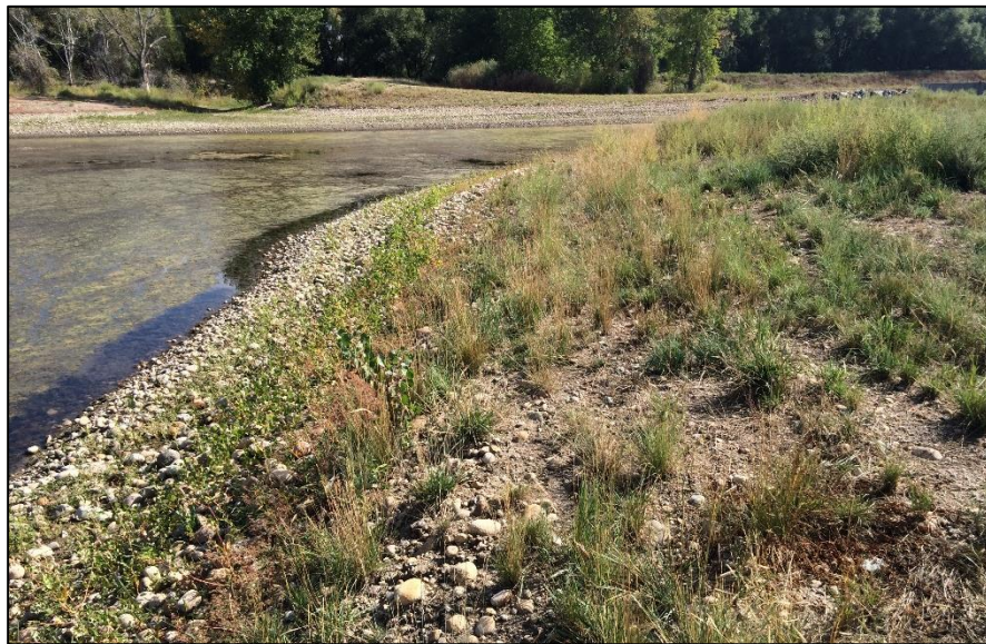
Photo 32. View of southern shoreline of pond 6 in area south of river. Pond slopes are at 3H:1V or flatter with good vegetative cover.
