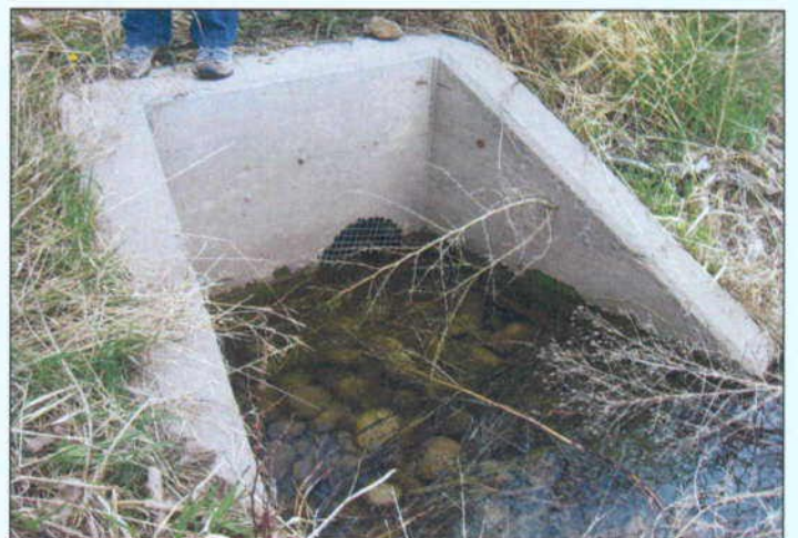
4. Clay-lined pond outfall on St. Vrain River.
