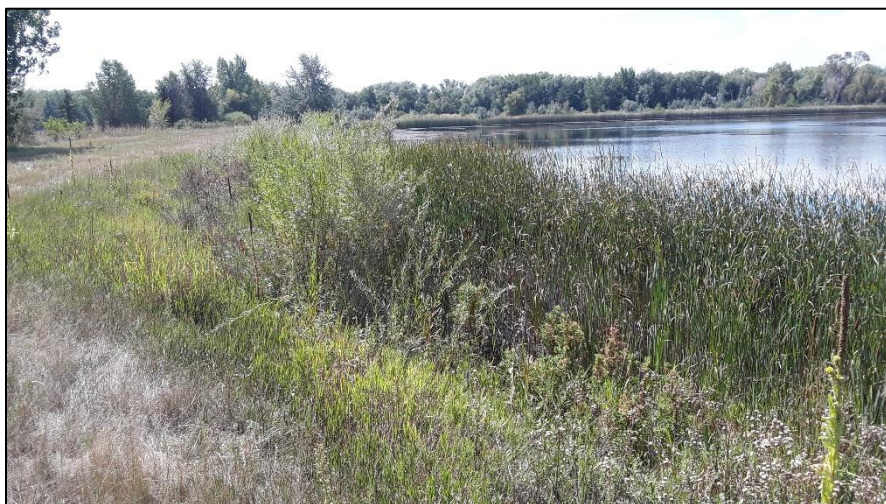
Photo 6. View of northeastern shoreline of east pond in area north of river. Pond slopes are at 3H:1V or flatter with good vegetative cover.
