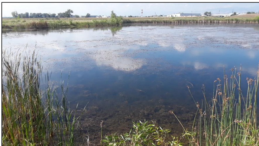
Photo 36. View of northern shoreline of pond 7 in area south of river. Pond slopes are at 3H:1V or flatter with good vegetative cover.
