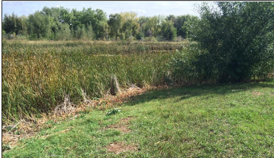
Photo 16. View of southeastern shoreline of pond 1 in area south of river. Pond slopes are at 3H:1V or flatter with good vegetative cover.
