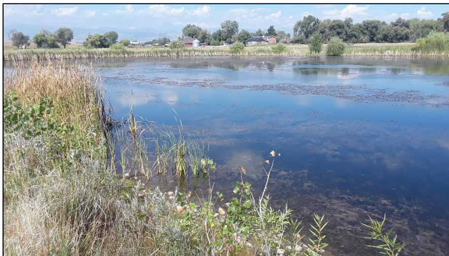
Photo 21. View of southern shoreline of pond 3 in area south of river. Pond slopes are at 3H:1V or flatter with good vegetative cover.
