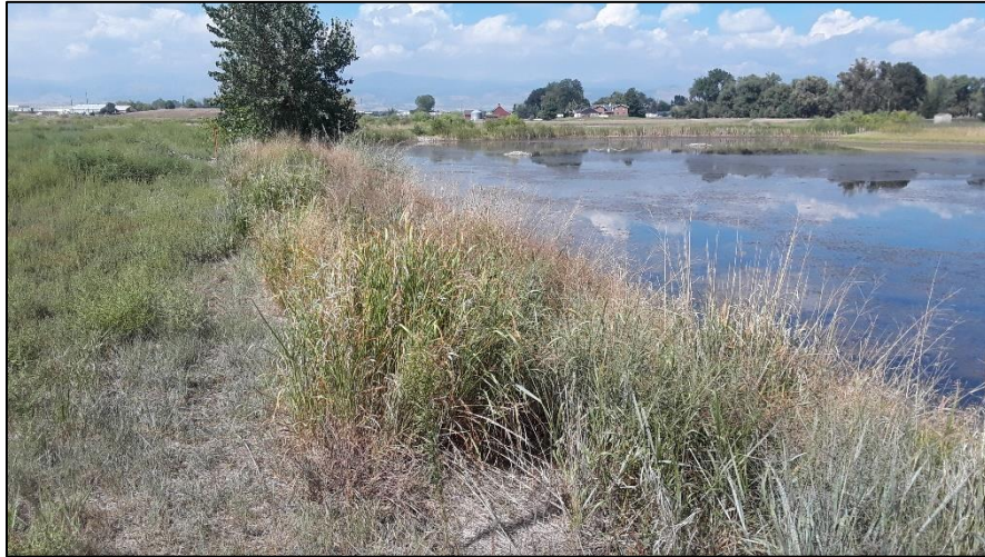
Photo 25. View of southern shoreline of pond 4 in area south of river. Pond slopes are at 3H:1V or flatter with good vegetative cover.
