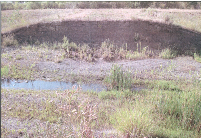
3. Breach between sediment pond and easternmost pond.
