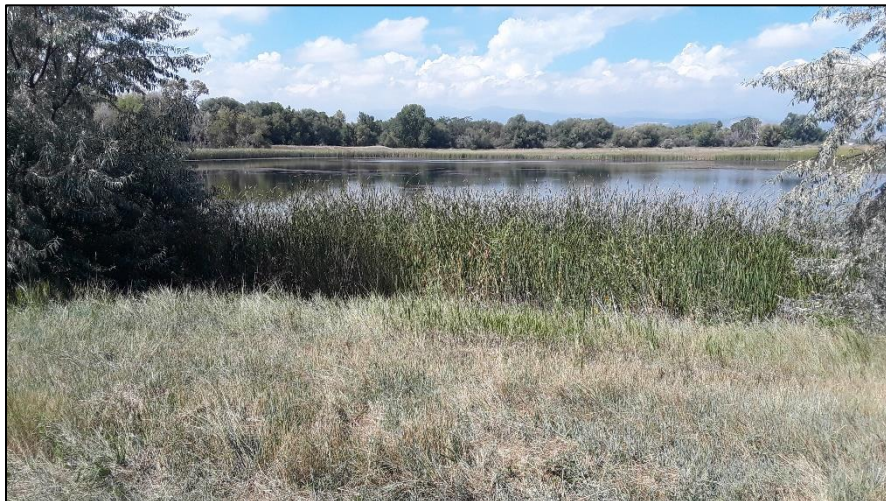
Photo 5. View of eastern shoreline of east pond in area north of river. Pond slopes are at 3H:1V or flatter with good vegetative cover.
