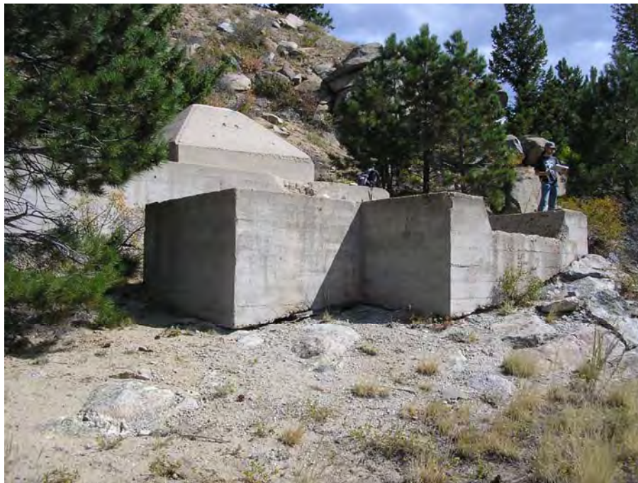
Figure 5-12. Cableway No. 1 foundations (Feature C) at Gross Dam and Reservoir, looking ESE.
