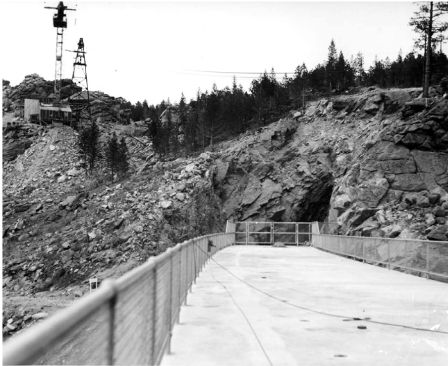
Figure 5-11. Historic photo (5/21/1955) of Cableway No. 1 and Cableway No. 2 features (Feature C). Note the building complex at the base of the headtower (left), which is taller than the tailtower (right) (Photo from the archives of Denver Water).
