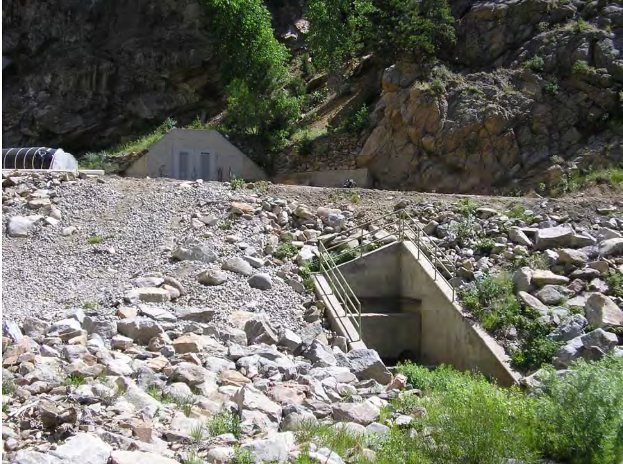
Figure 5-14. Photo of outlet works, looking NE. Entrance to valve chamber access channel is visible near top of photo; more recent (1970s) outlet in foreground.
