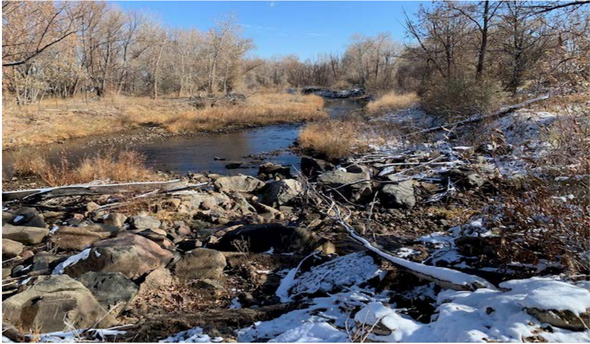
Looking east from the existing diversion structure into the phase 2 area.
