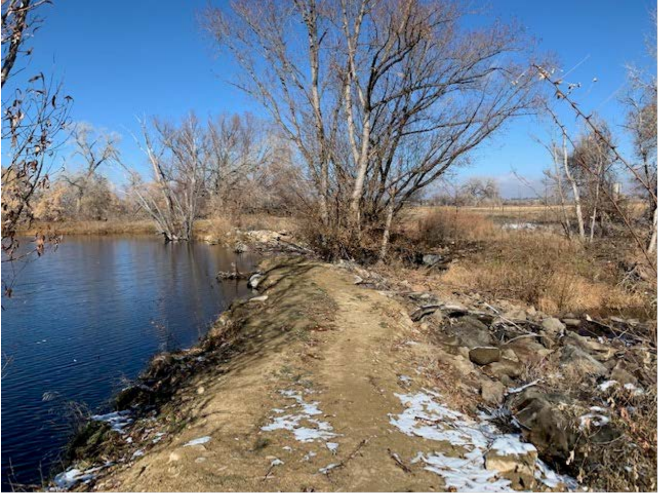
The existing diversion structure
