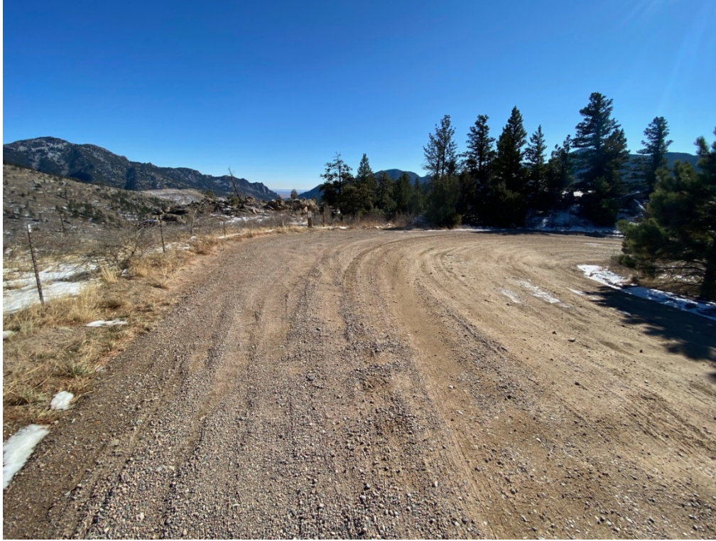
Figure 9 Example of widening of a curve on Gross Dam Road to accommodate turns by larger hauling trucks.
