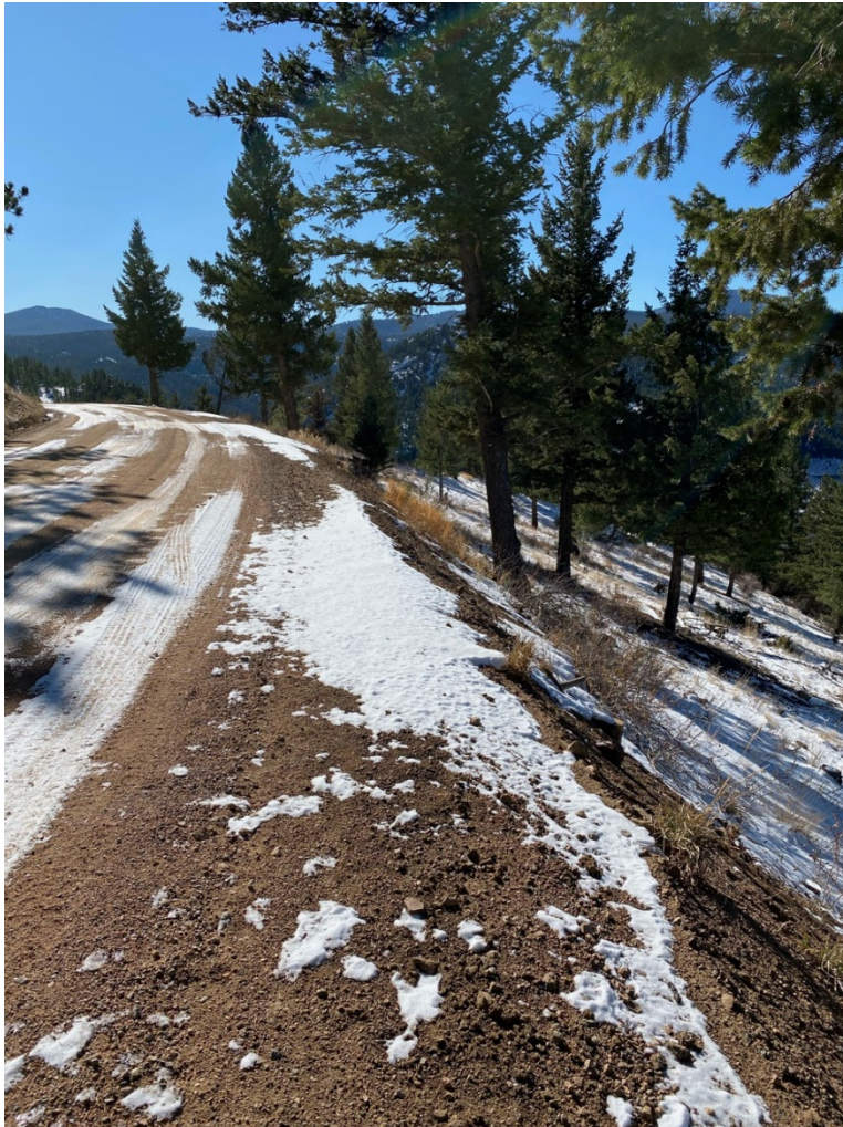
Figure 8 Example of road widening along Gross Dam Road. This type of expansion can be found all along the road.
