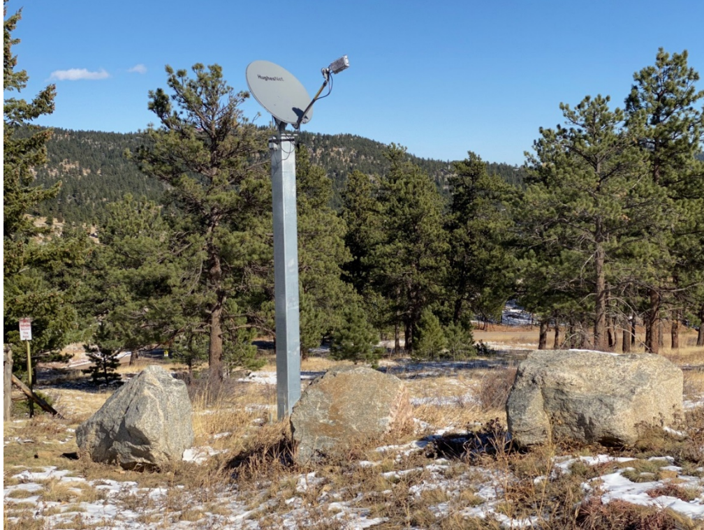
Figure 12 New communications satellite installed for monitoring transmission line from the Gross Dam Hydro Power plant.
