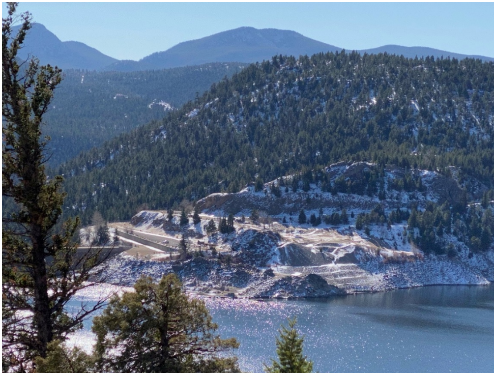
Figure 1 Expanded staging area at south end of dam, viewed from the North Shore. Also visible is the new terracing on the face of old quarry used for the original dam construction.
