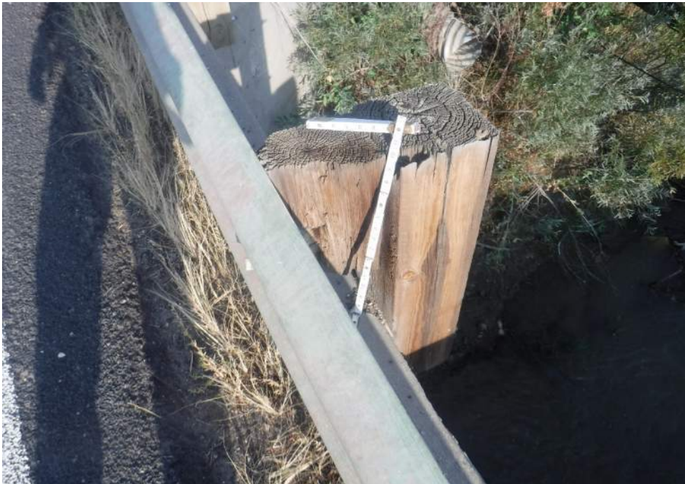
SPLIT SPACER BLOCK AT 2ND POST FROM WEST IN NORTH RAIL
