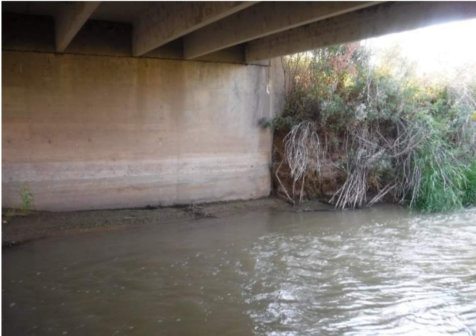
BANK EROSION AT SOUTHEAST CORNER
