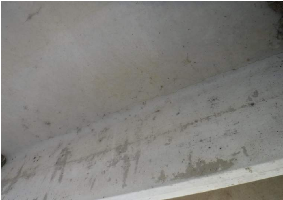
TYPICAL CRACKS UP TO 0.09 INCHES WIDE IN GIRDER FILLETS
