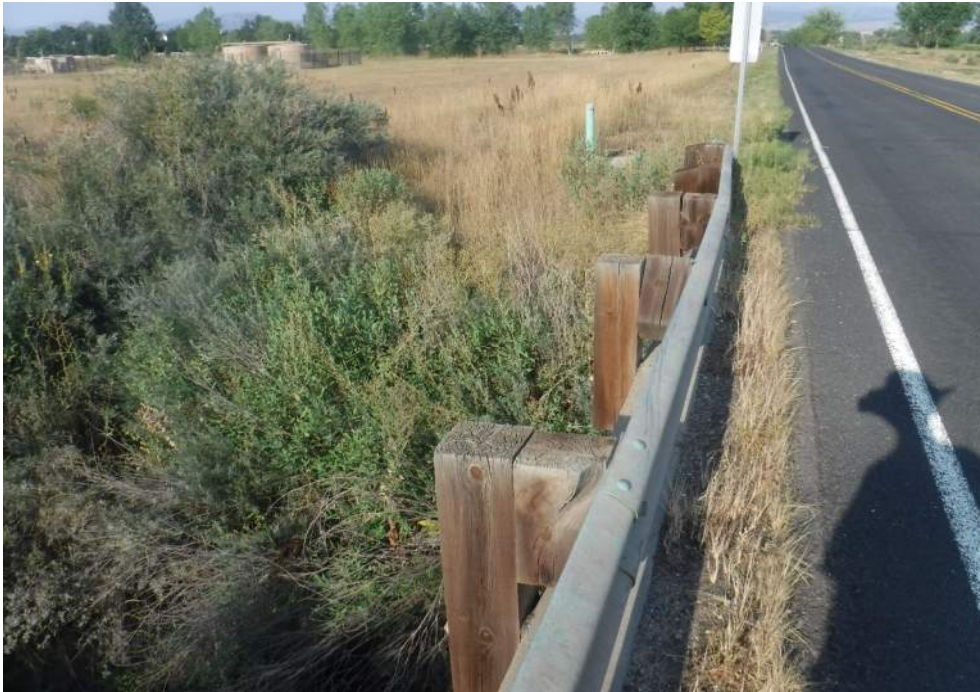
TWISTED SPACER BLOCKS IN SOUTH RAIL
