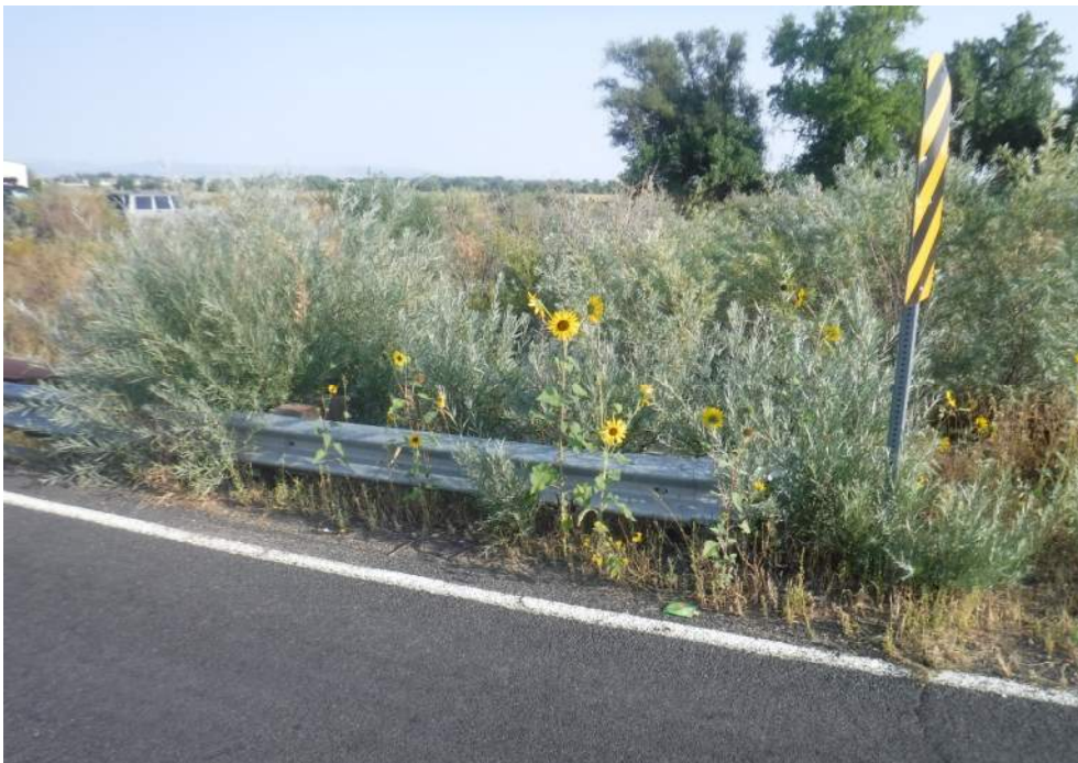
HEAVY VEGETATION AT NORTHEAST APPROACH RAIL
