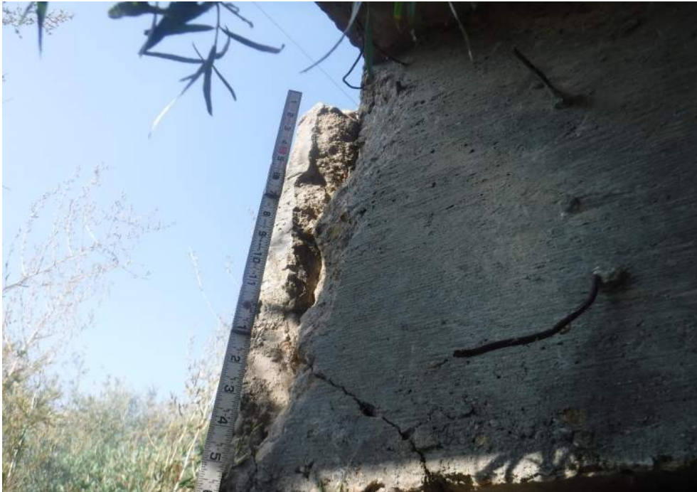
21 INCH LONG X 4 INCH WIDE X 1 INCH DEEP SPALL IN JOINT OF SOUTHWEST END DIAPHRAGM
