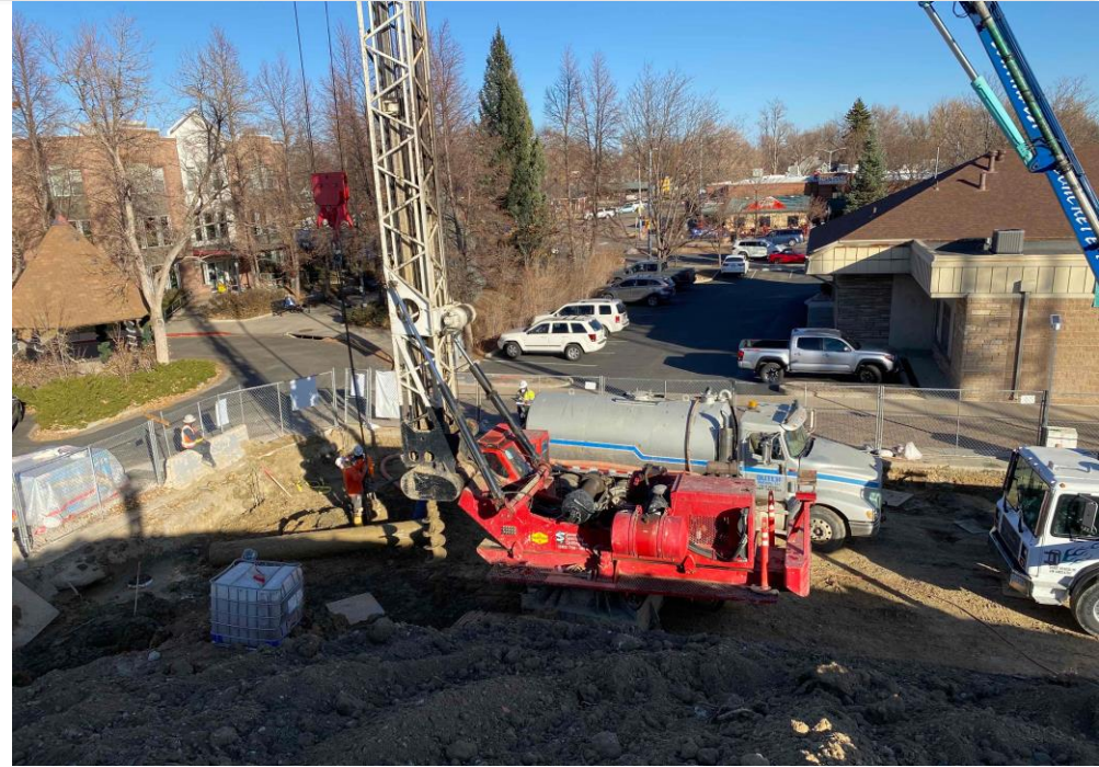
View of the northeastern side of the residential site. Drill rig boring into bedrock
