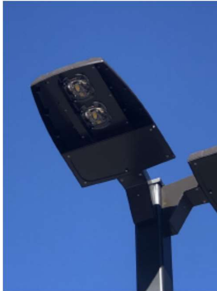
Upgraded high pressure sodium lighting to LED lighting saving energy and cost.
