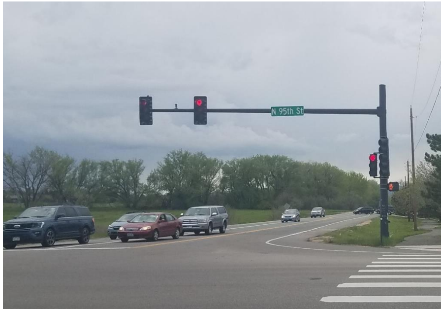
Signal Pole w/ Mast Arm (N 95th Street and Niwot Road)
