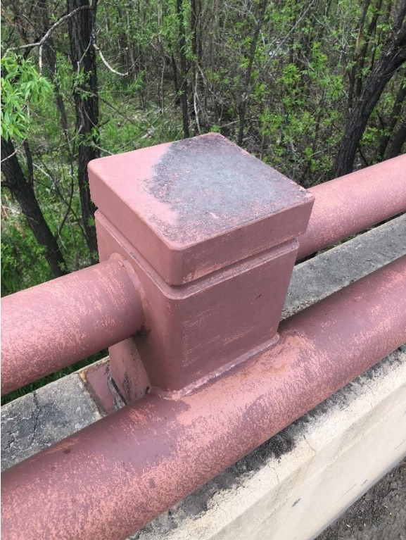
Details of chipping, corrosion and weathering of posts and post/rail interface.
