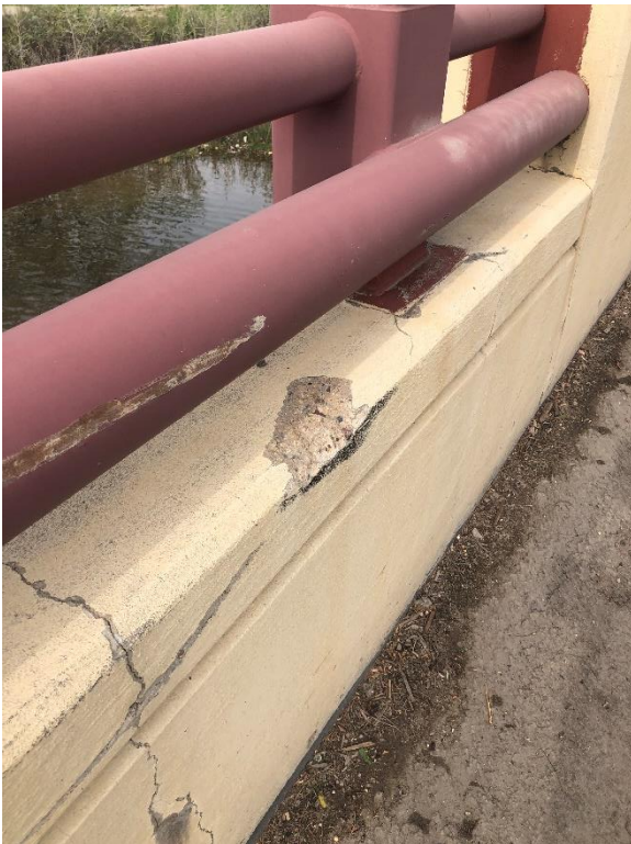
Details of chipping, scrapes, corrosion and weathering of posts, rails, and post/rail interface.
