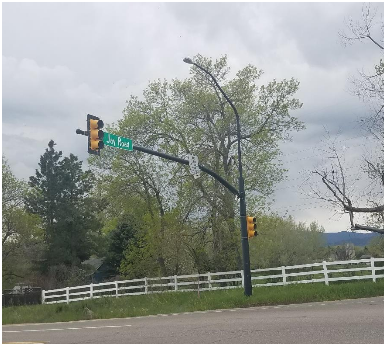
Signal Pole w/ Mast Arm and Luminaire Arm (N 75th Street and Jay Road)
