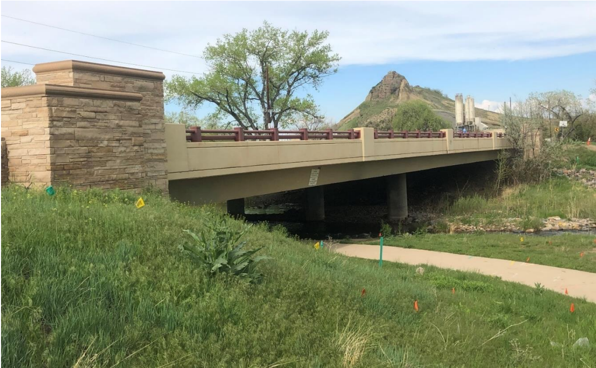
Current photo of bridge
