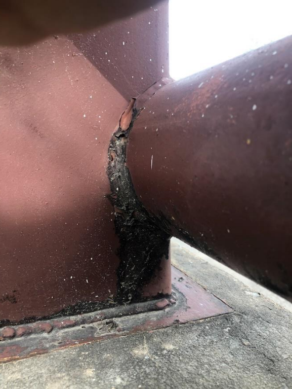
Details of chipping, corrosion and weathering of posts and post/rail interface.
