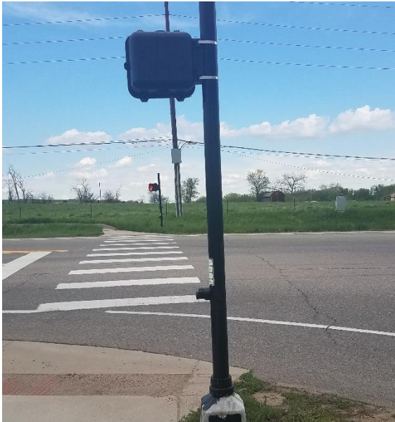
Ped Poles (N 75th Street and Jay Road)
