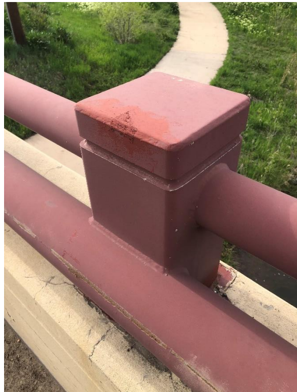
Details of chipping, scrapes, corrosion and weathering of posts, rails, and post/rail interface.
