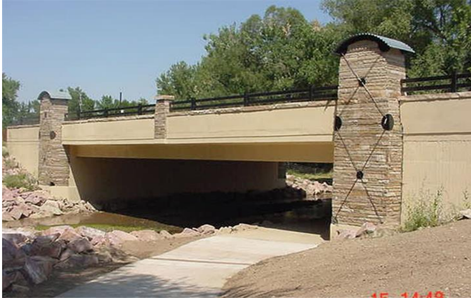
Photo of bridge (circa 2004) showing bicycle rails and decorative ironworks on pilasters
