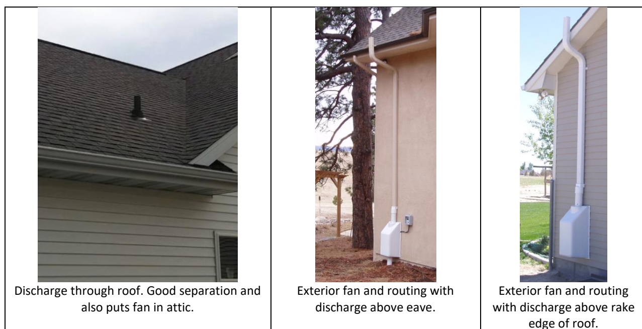
Figure 66: Proper Discharge Points
