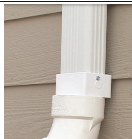
Figure 63: Adapting exterior pipe to downspout
