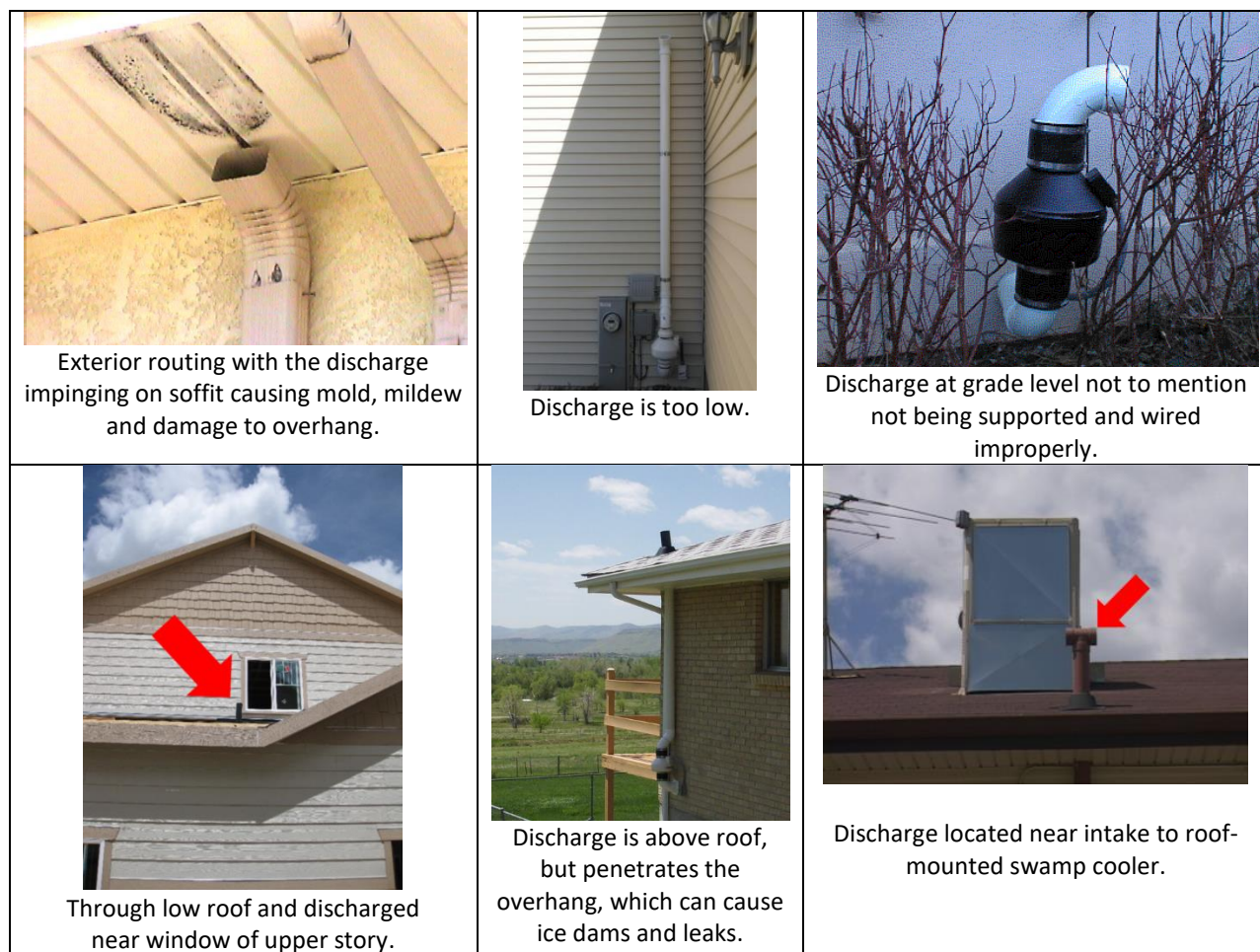
Figure 67: Improper Discharge Points
