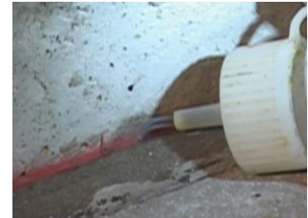
Soil depressurization reverses air flow direction. Air goes DOWN rather than UP through foundation.
