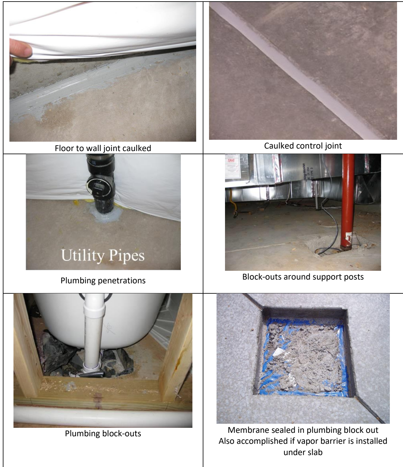
Figure 75: Slab Caulking and Sealing Examples
