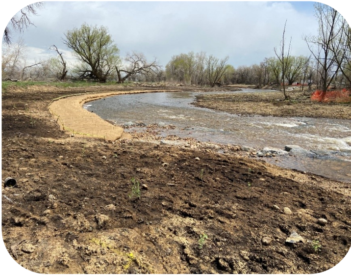
Niwot Ditch Fish Passage: After dam removal, the creek was reshaped into a natural channel and used buried boulders instead of concrete to divert decreed water rights.
