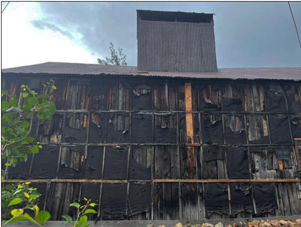
Figure 36. Photograph of Rocky Mountain Mammoth outbuilding in 2021.
