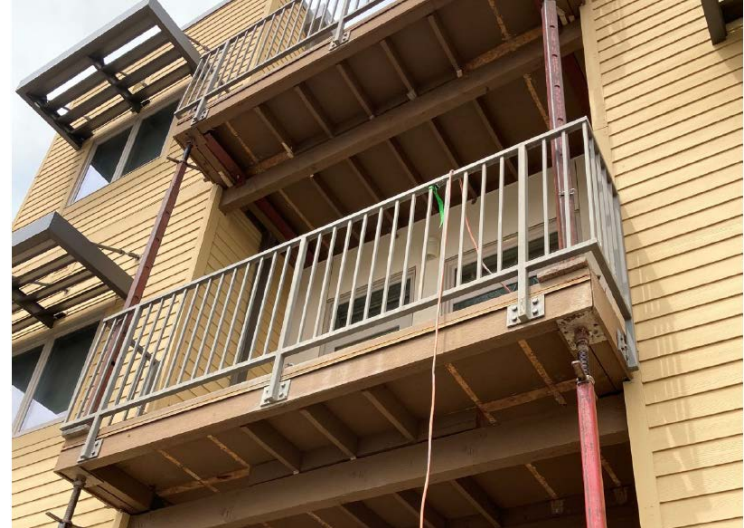
Decking cracked and shifted due to twisting & weathering of support beams
