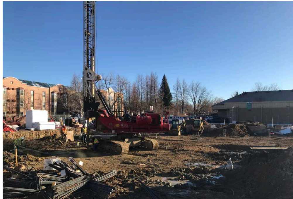
View of the northeastern area of the residential site. Drill rig boring into bedrock
