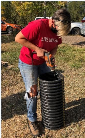
Drilling holes at cross sections of culvert pipe.
