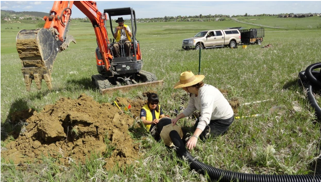
Installing an artificial burrow after digging a trench.
