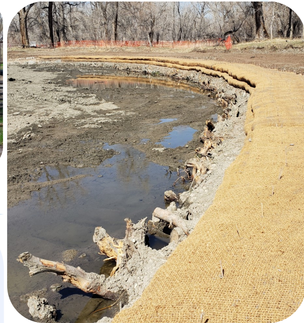
Above: toe wood structure #1, the same feature as pictured in the top photo, after construction is completed. Willow stakes are anchored into the two soil lifts and will soon take root and fortify the feature.
