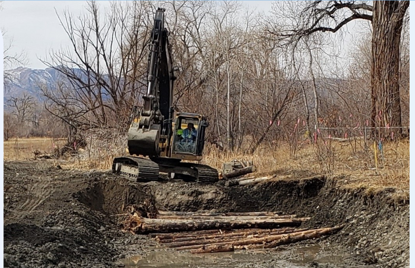
Above: An excavator carefully places logs at an outer bend of the St Vrain Creek as a part of the Niwot Ditch Diversion Project. The outer section of this row of logs will be covered with slash and fill material before being covered with riparian seed-laden soil lifts that will be supported with hundreds of willow stakes. This toe wood structure provides a strong natural barrier that protects the channel from erosion and provides fish habitat.
