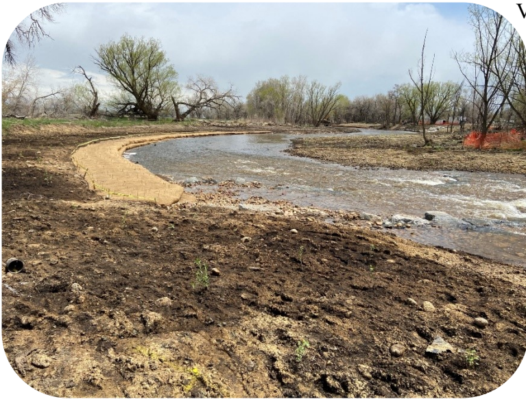
Niwot Ditch Fish Passage: After dam removal, the creek was reshaped into a natural channel and used buried boulders instead of concrete to divert decreed water rights.
