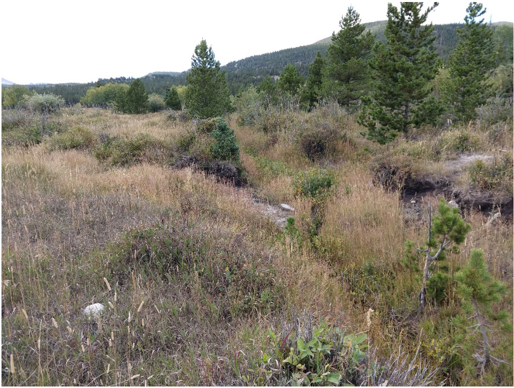
Lower section of main ditch; August 21, 2020. Looking west below Point A.
